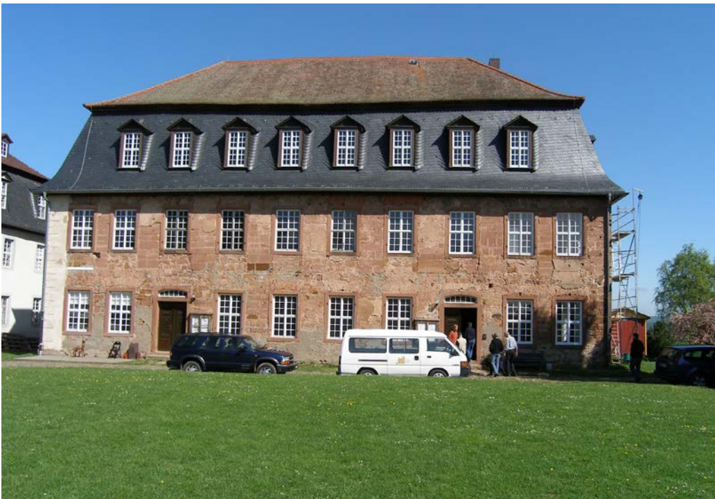
3.49 Grafenhaus in Herrnhag, built 1744. The shape of the roof can be recognized in other moravian settlement, primarily in the central european area.
