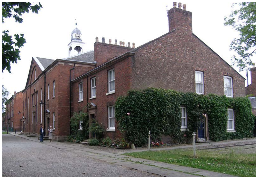
3.47 The church in Fairfield is influenced by English building culture, yet the spire is a recognisable element.
