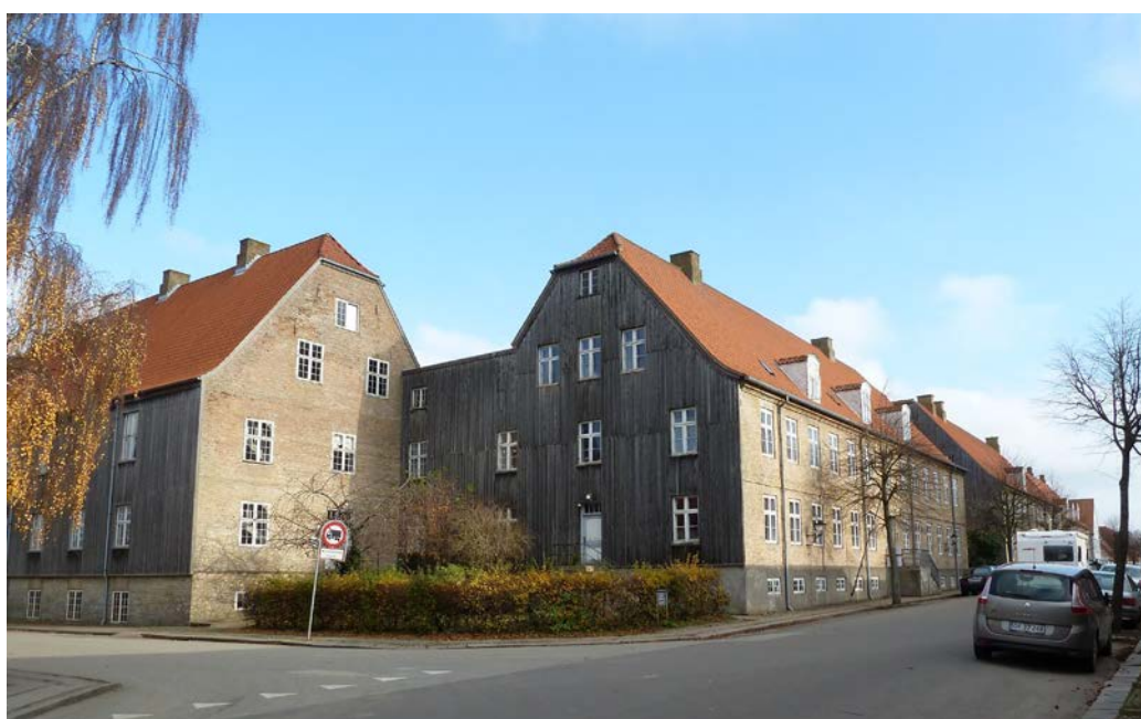
2.28 Facade of the Widow House facing Nørregade and Birkevej. The western-facing gables are board-clad, while the other facades are brick.
