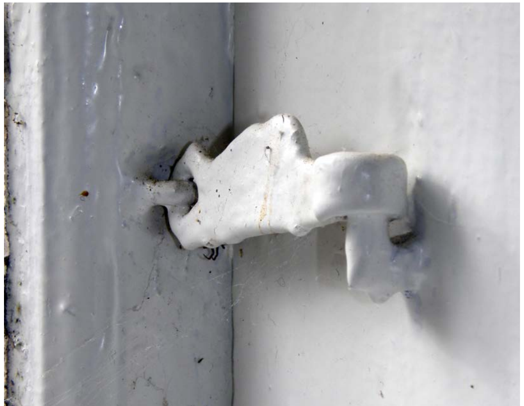
2.31 An example of preserved older casement fasteners on a window.
