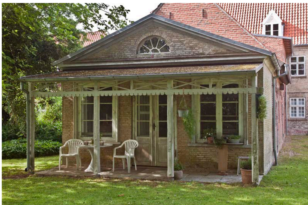
2.40 Pavilion to Lindegade 24. There are several examples of this type of pavilion in the town. The pavilion is built onto a side building of the property and a half-roof forms a room in front of the pavilion facing the garden.
