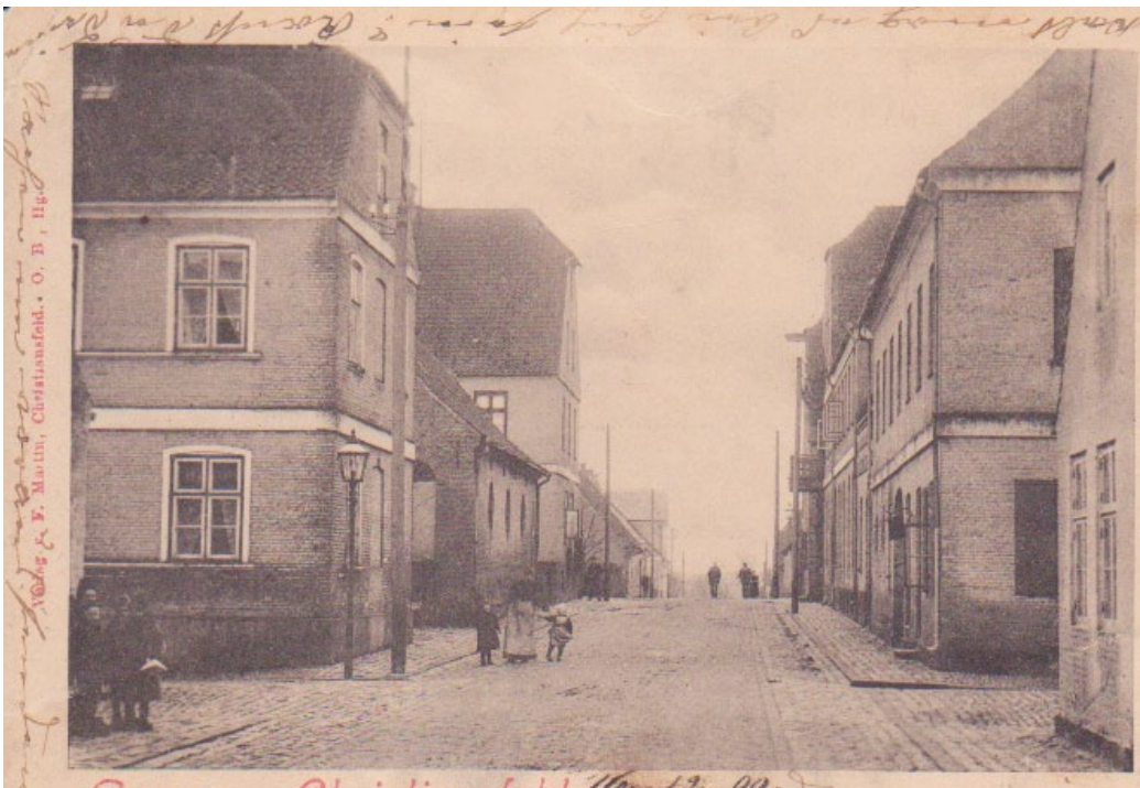
2.70 Postcard showing Kongensgade seen to the south from the junction at Nørregade. Undated (Local History Archive).
