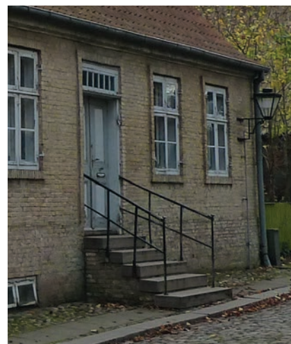
Illustration 7 - Nørregade 7 example of front door with granite staircase and wrought-iron railings.
