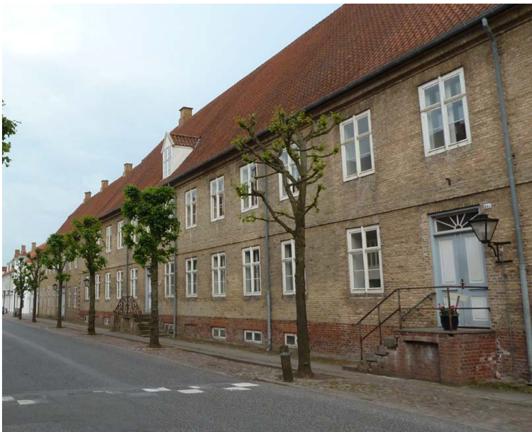
2.26 The facade of the Brothers' House onto Lindegade. The facade is elongated and there are several entrances.
