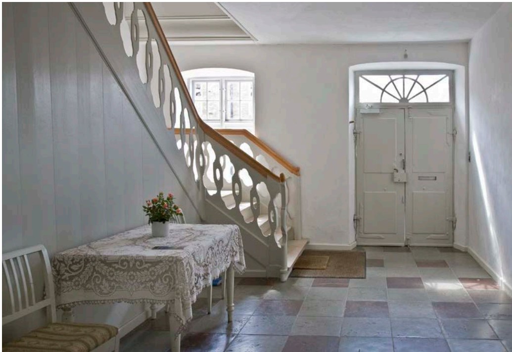
2.15 Staircase in the Widow's House, Lindegade 16. There are many parallels to other Moravian towns in the design of stairs and stairwells in Christiansfeld. The Baroque design is distinctive and is seen in several buildings. The floor here is covered with Öland stone, a material that is connected with the region and is seen in many older buildings in Denmark, but not in other Moravian towns.
