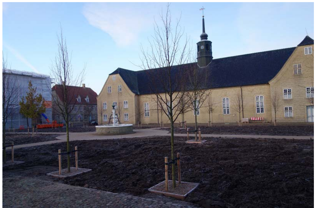
4.1 The Church Square during the current renovations. At this point new linden trees have been planted and the paths have been established.
