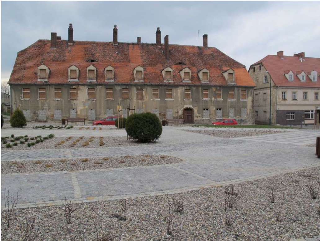
3.48 Building in Gnadensfrei. The body of the building is recognisable, with its depth, steep roof, small gable, and numerous attic rooms. Unfortunately, it has been very poorly maintained.
