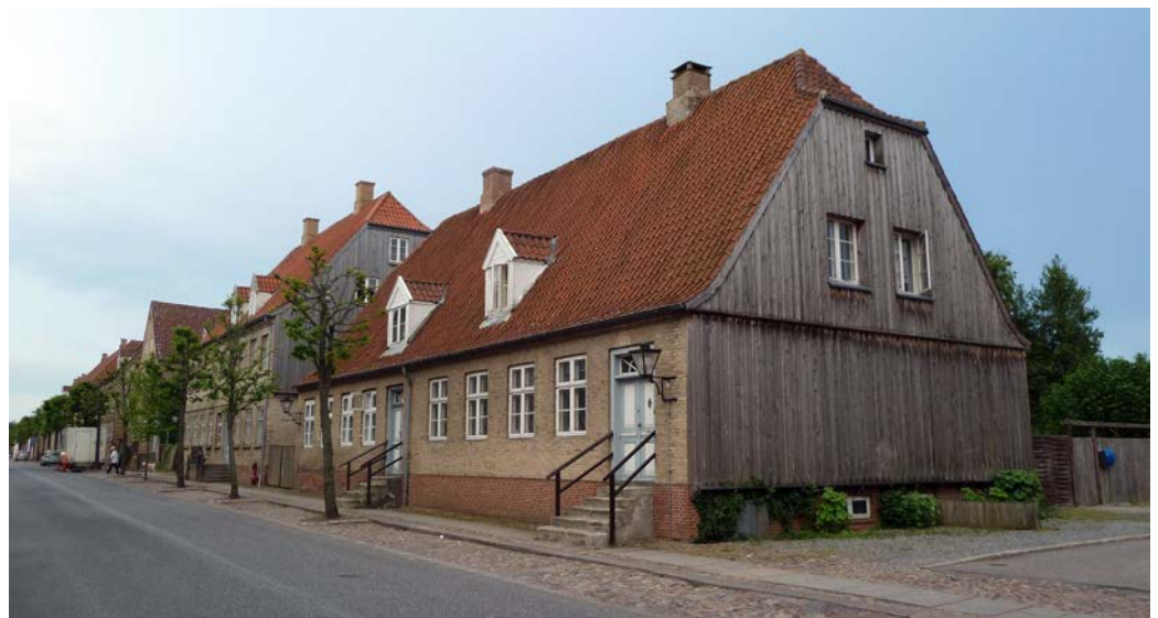
2.17 Lindegade 20 and 22, which are two adjoined family houses. At the back the two storeys of Lindegade 24 can be seen. Both buildings have distinctive steep tiled roofs and quarter-hipping, which is characteristic of the architecture in Christiansfeld.
