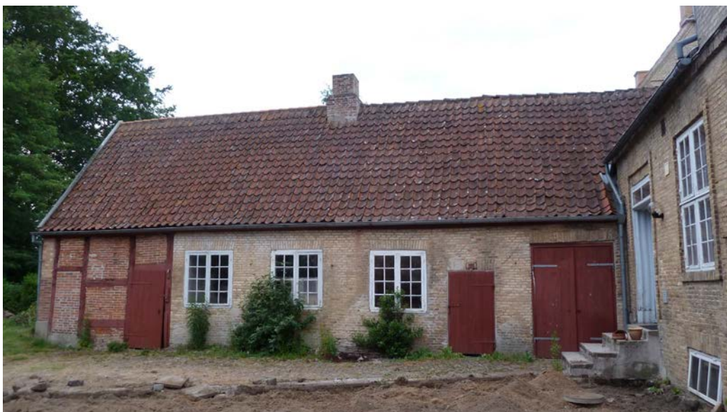
2.36 The western side house of the Vicarage, which is adjoined to the front building. The southernmost part of the building is constructed in half-timbering, with central blocks in red brick.
