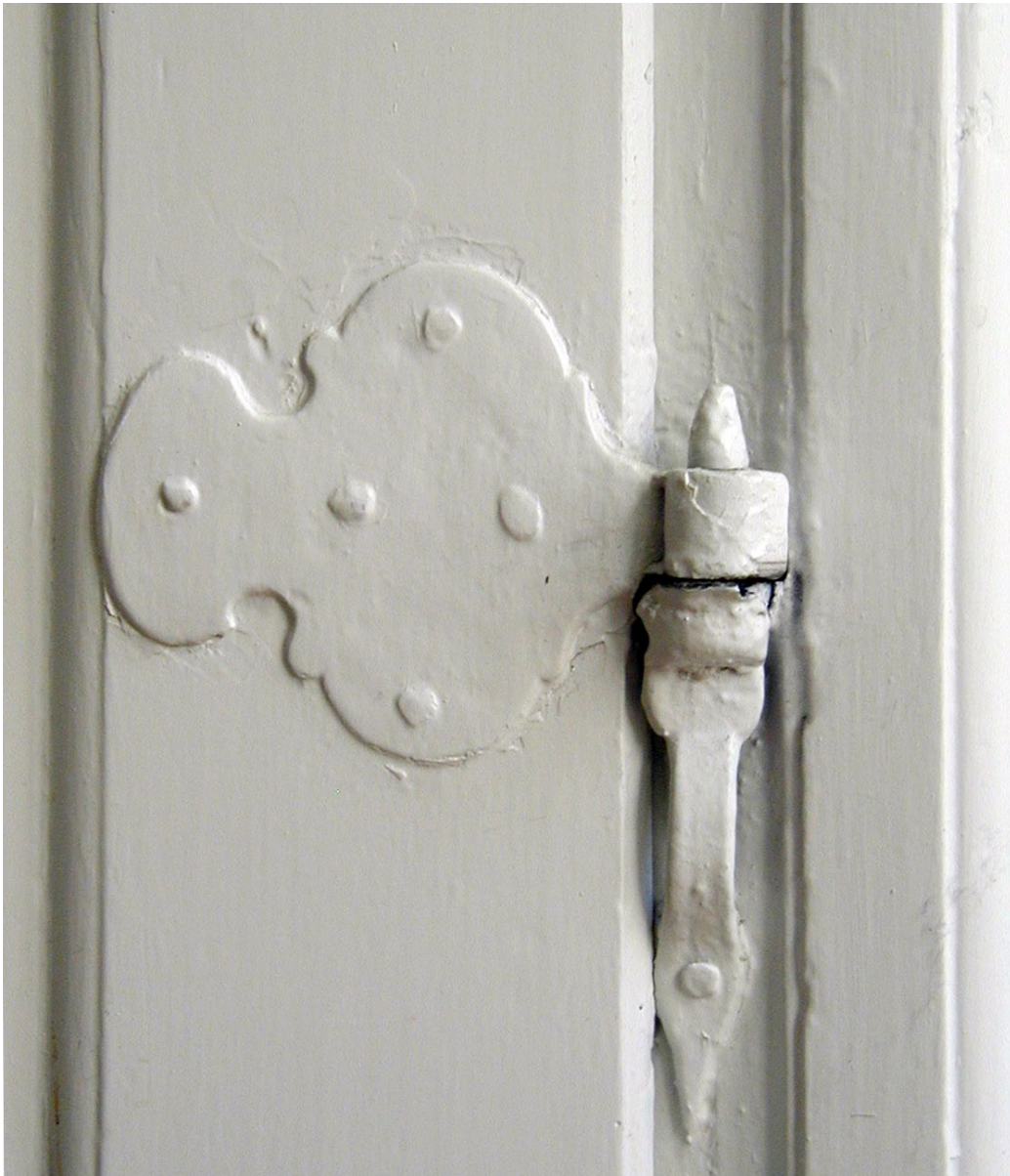
2.18 Wrought-iron hinge from a door in the Sisters' House, Nørregade 14. A typical example for Christiansfeld of an architectural detail and the quality of craftsmanship.
