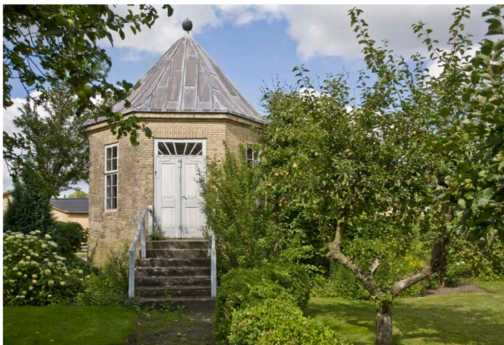
2.39 Garden house in the garden of the Widow House, Nørregade 16. The garden house is located at the end of the garden's central axis. This garden house is distinctive with its octagonal floor plan, walls of yellow brick and pointed rotunda roof.
