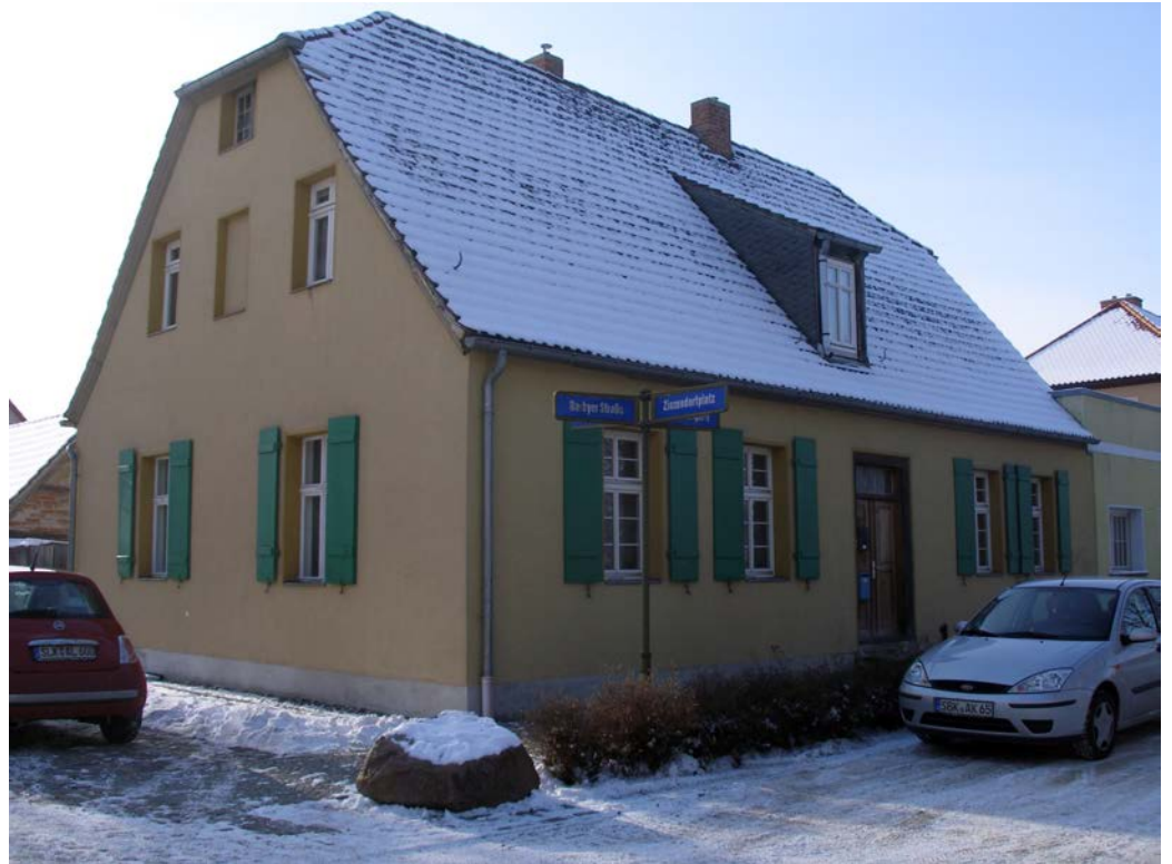
3.50 House by the church square in Gnadau, built 1771.
