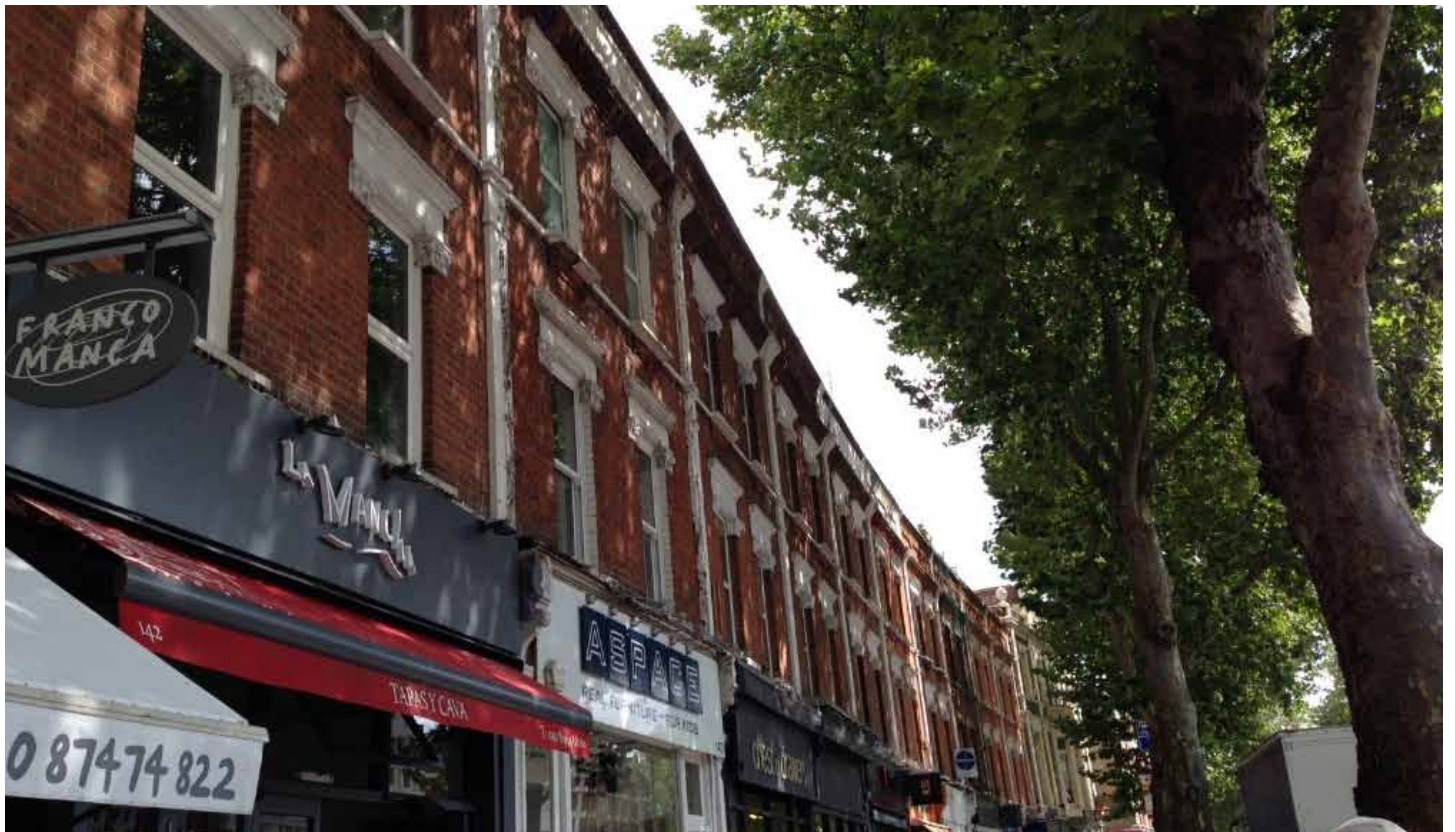
Figure 11: 148-178 Chiswick High Road, strong parapet line and regular fenestration pattern. January 2015
