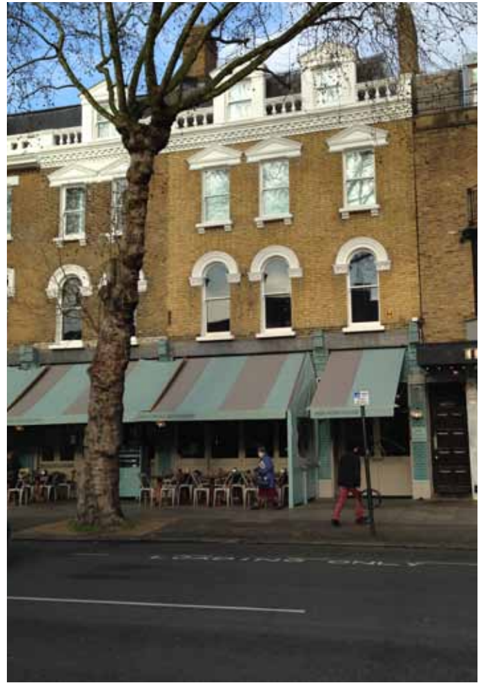
Example of original detailing Chiswick High Road
