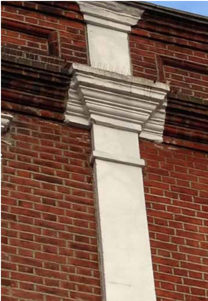
Example of pilaster and cornice detail on Chiswick High Road
