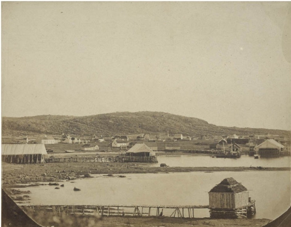
Figure 25. (t) Historic stages at the rooms of Southwest Crouse, 1857-9. Note how the pier of the stage serving the room (EfAx-10) at the bottom of the bay extends into the water to reach sufficient depth for landing chaloupes (Paul-Émile Miot Collection, LAC, PA-188223). (b) Detail of fishing stages at Croque Harbour at low tide, 1857-9 (Paul-Émile Miot Collection, LAC, PA-188225).
