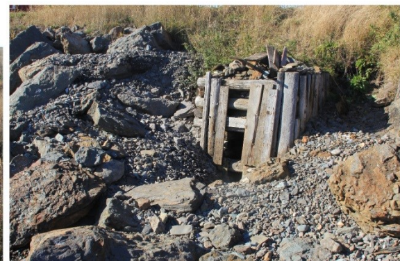
(F). A culverted spring, between two rocky outcrops, separated two rooms in Southwest Crouse.
