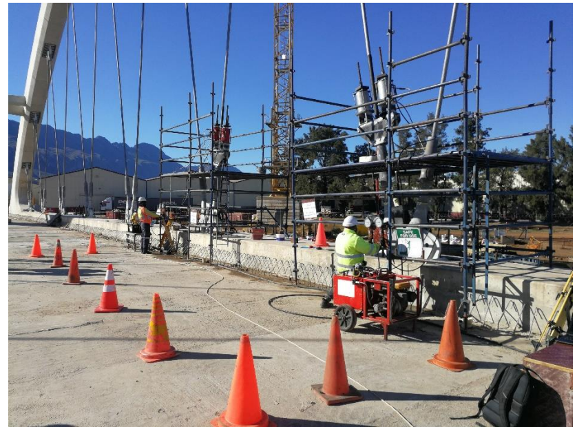
Simultaneous tensioning of 2 cables per Arch
