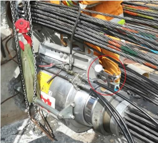
Figure 49 Jack with magnetic precision Dial Gauge
