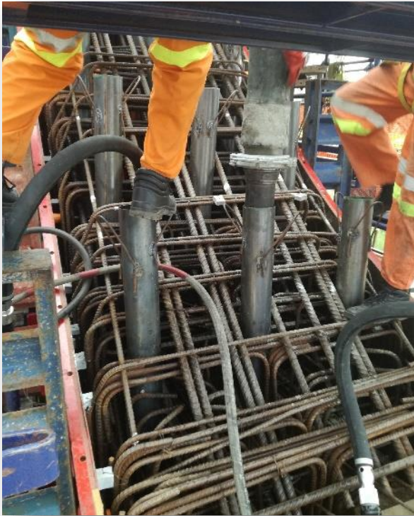
Steel tube concrete pour access provided through congested reinforcement
