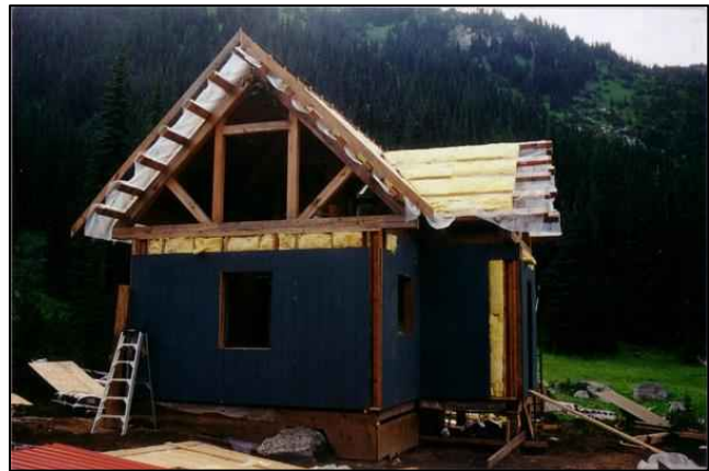
The Hut under construction in 1998.
