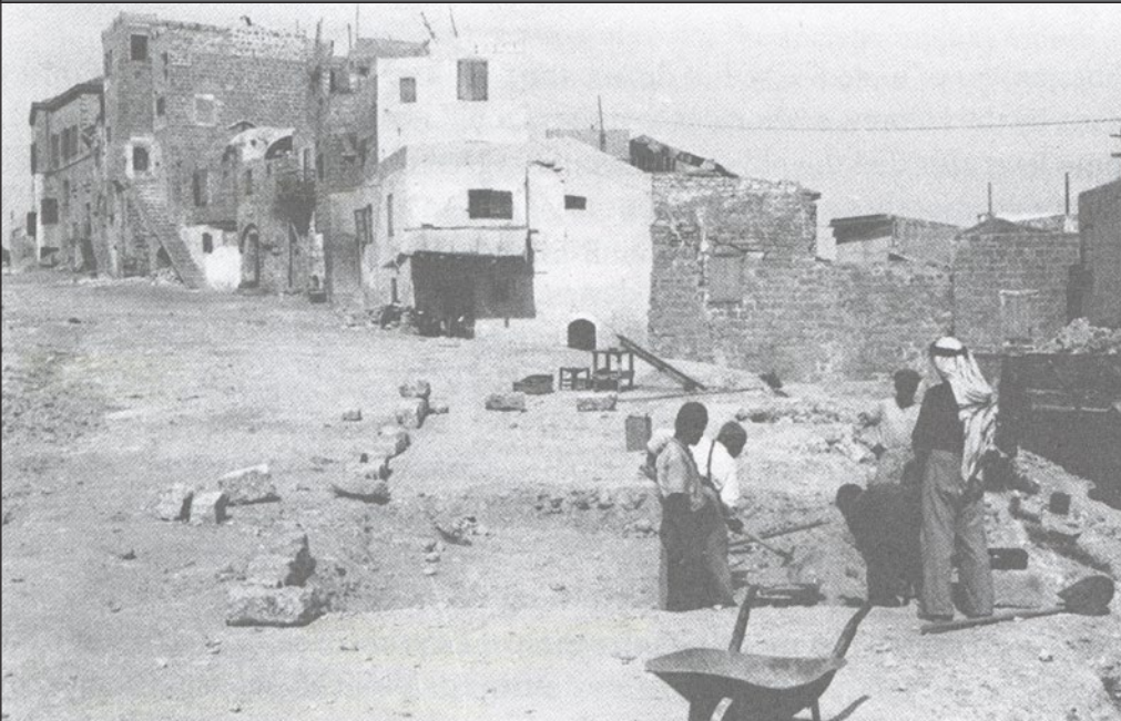
Photo 4.2: Excavating Destroyed Jaffa Neighbourhood
