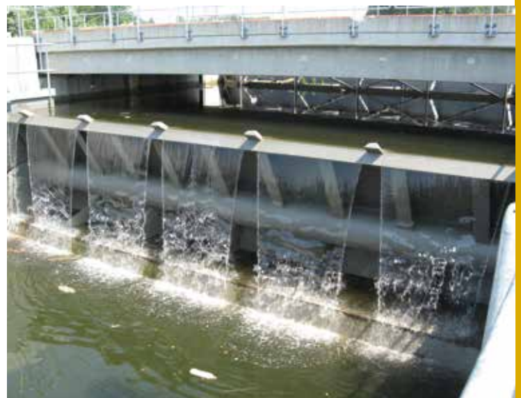
Steel construction + Electromechanical equipment of weir at Lock Asper (Belgium)
