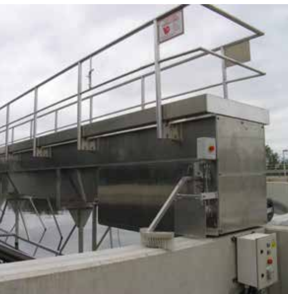
Scraper bridge Aluminium Profile - tank diameter 42,5 m - RWZI Harelbeke (Belgium)
