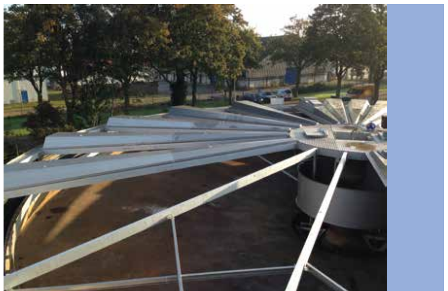
Scraper bridge with rotating roof in Aluminium - diameter tank 27 m - Dronten (Netherlands)
