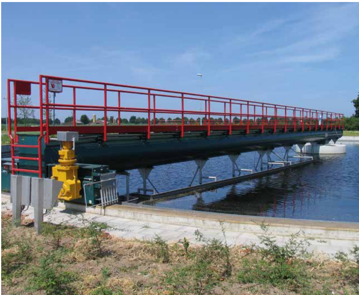
Scraper bridge - steel tube construction - tank diameter 48,5 m - Aarle Rixtel (Netherlands)
