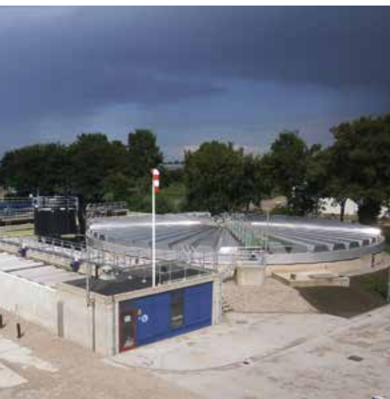
Scraper bridge with rotating roof in Aluminium - diameter tank 27 m - Dronten (Netherlands)
