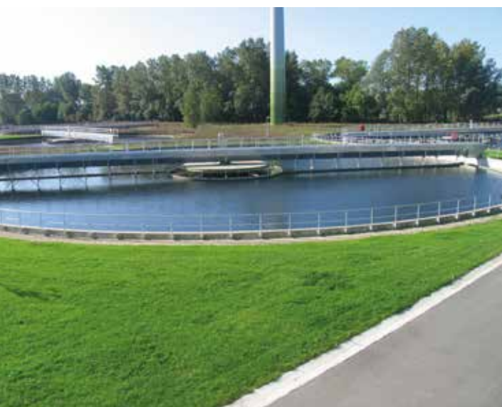
Scraper bridge Aluminium Profile - tank diameter 52 m - RWZI Brugge (Belgium)
