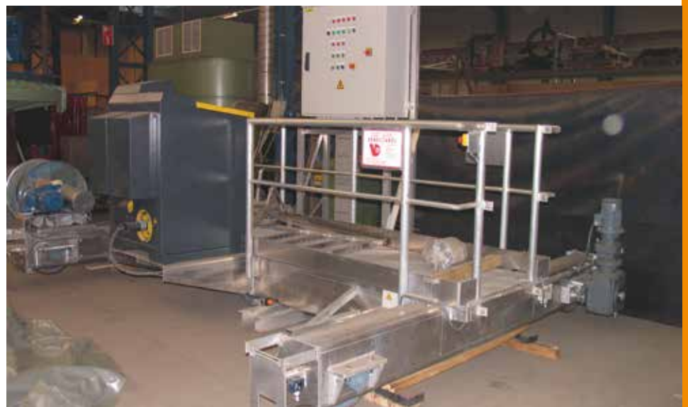
Construction of gantry unit
