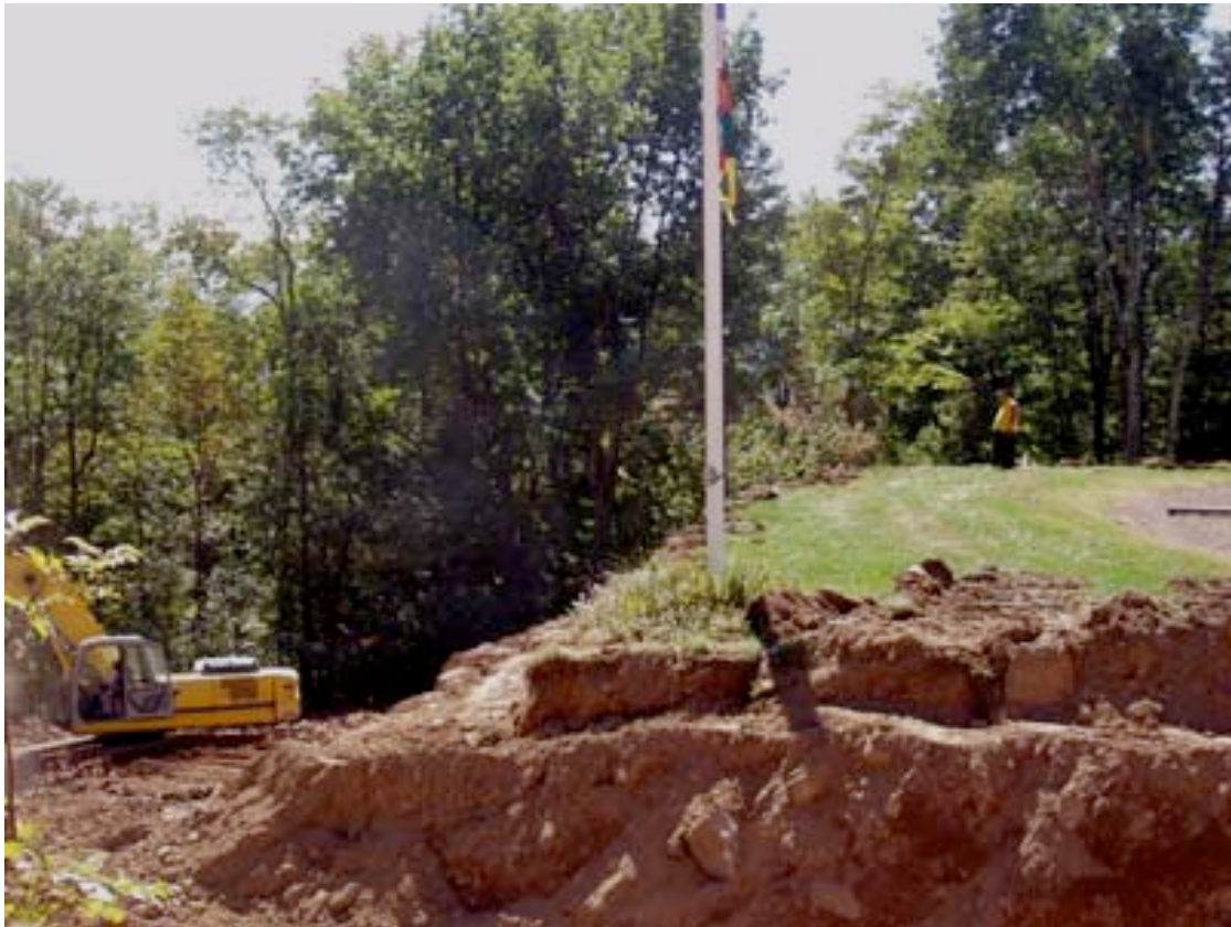
Figure 9: Construction underway, KTD
