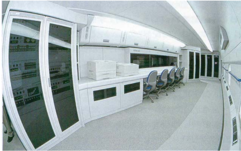
Figure 4: Measurement room of track inspection car in T4
