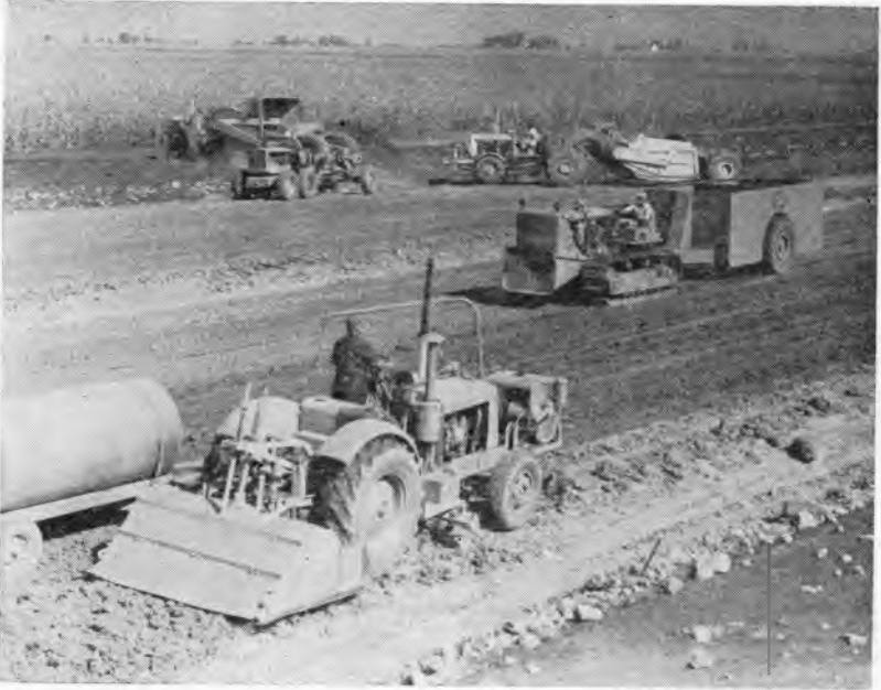
Fig. 2. Four types of equipment played major roles in the grading phase of the AASHO Road Test construction. Shown here are a rotary speed mixer (foreground), a pneumatic compactor (right center), and a blade grader and two earth movers (background).
