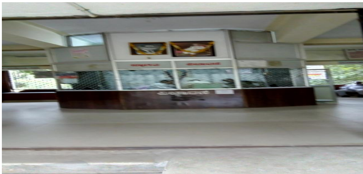
Pic. 10. Gulbarga Mahanagar Palika (Non-functional Helpdesk)
