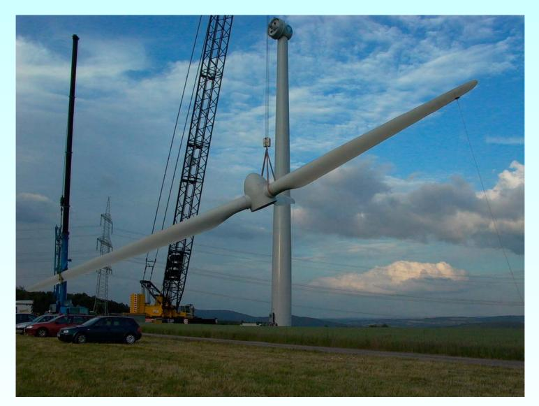
1.2 MW turbine wind rotor diameter 62 m pole height 69 m speed 21/min pitch control electrical pitch drives Nacelle and rotor mass: 81 t
