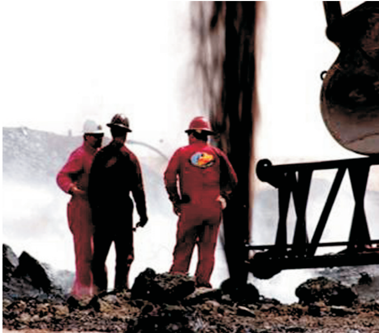
Boots & Coots personnel supervise the insertion of a stinger that would be attached to a Halliburton pump that delivered drilling mud, controlling the well pressure and killing the well.
