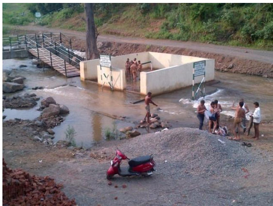
Hot Spring Bath(Under Construction)
