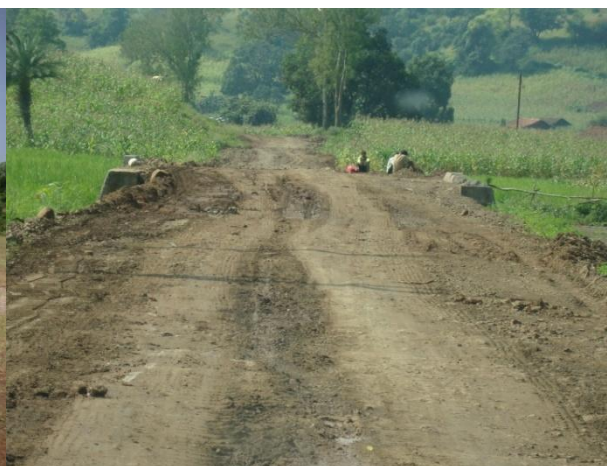
Access Road to Sita Khai
