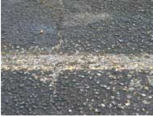
Figure 1. High Severity Wear Paint Lane Marking.
