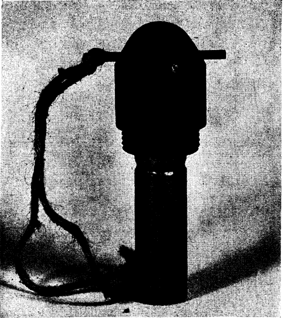
Figure 186.—Fuze for Type 3 (1943) conical hand-thrown mine, small size.
