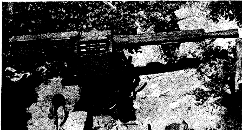
Figure 160.— Vickers 40-mm gun, single-mount.
