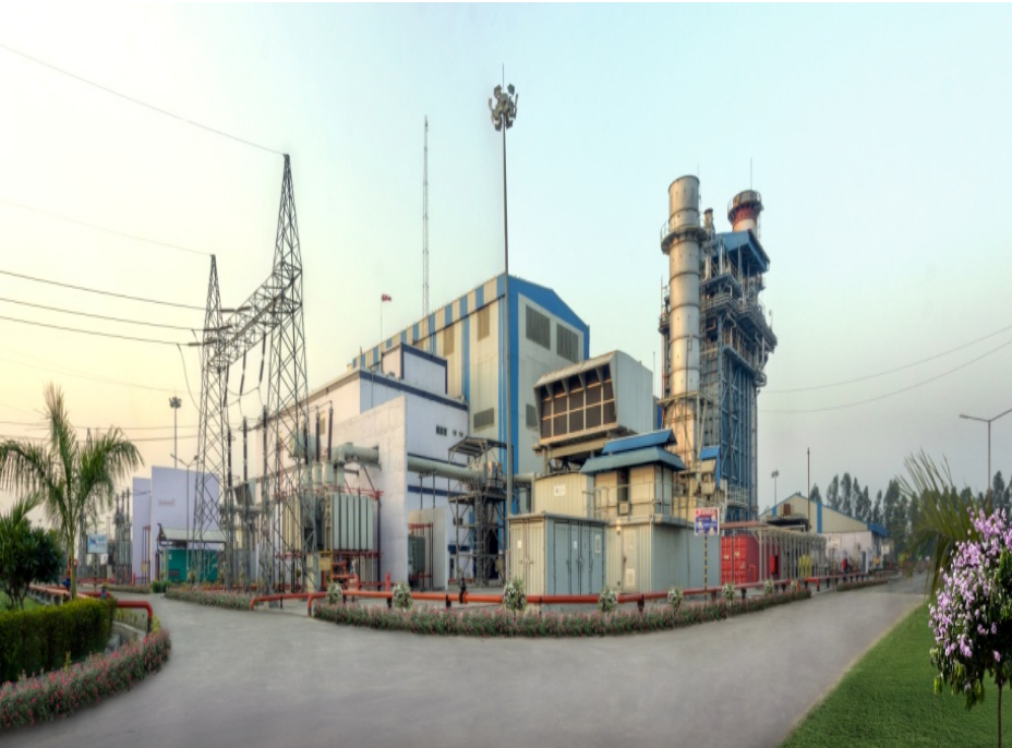
Kashipur gas based combined-cycle power plant, Uttarakhand, India
