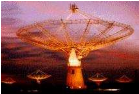
Figure 1: Giant Metrewave Radio Telescope (GMRT) near Pune, a radio interferometer consisting of 30 dishes of 45 m diameter each, spread over distances spanning \sim 30 km, is the world's largest radio telescope operating at metre wavelengths
