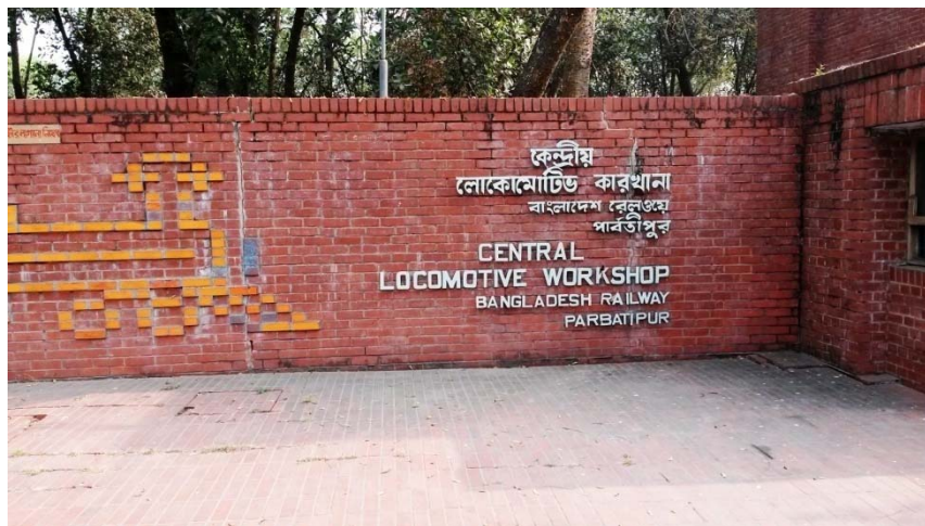
Figure 3-1: Entrance Gate Central Locomotive Workshop, Parbatipur
