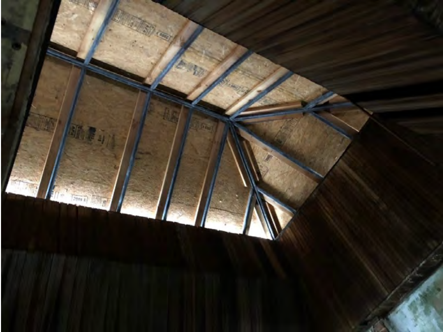
Photo 14, Looking up at roof skylight
