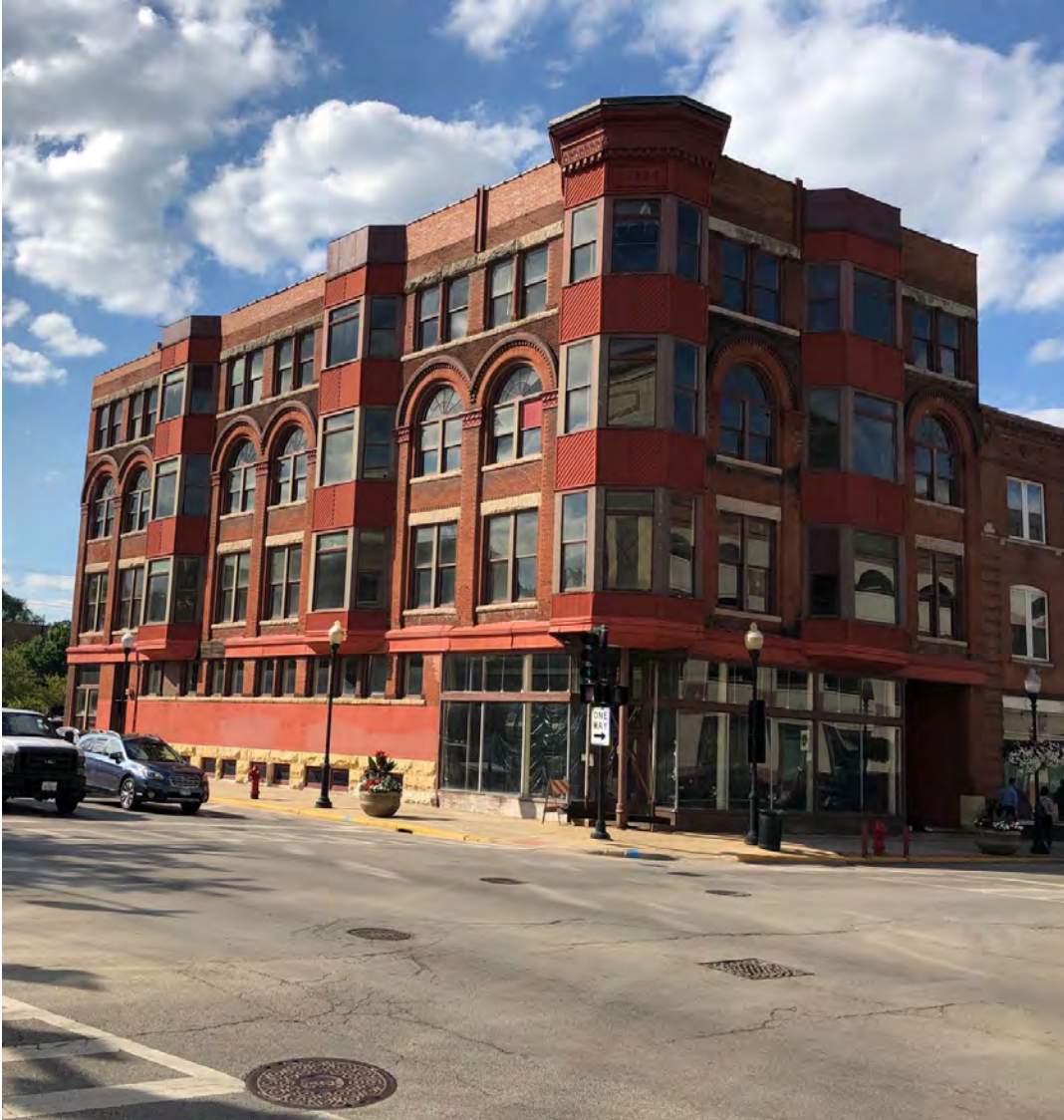
Photo 1, Primary (East) and South façade, looking NW
