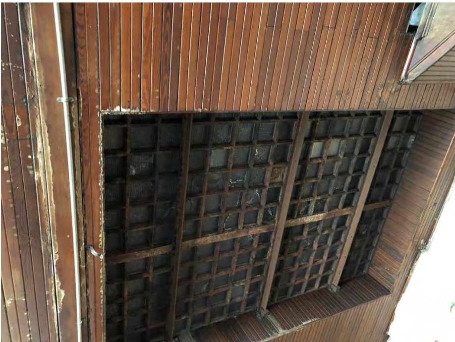
Photo 13, floor light between 3 rd and 4 th floor
