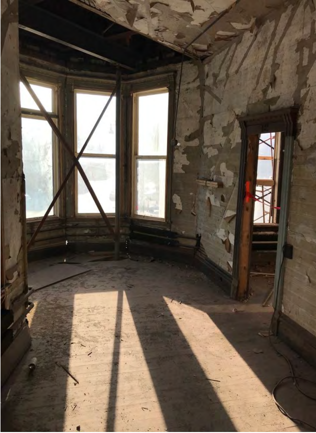
Photo 6, Turret 2 nd floor, looking SE
