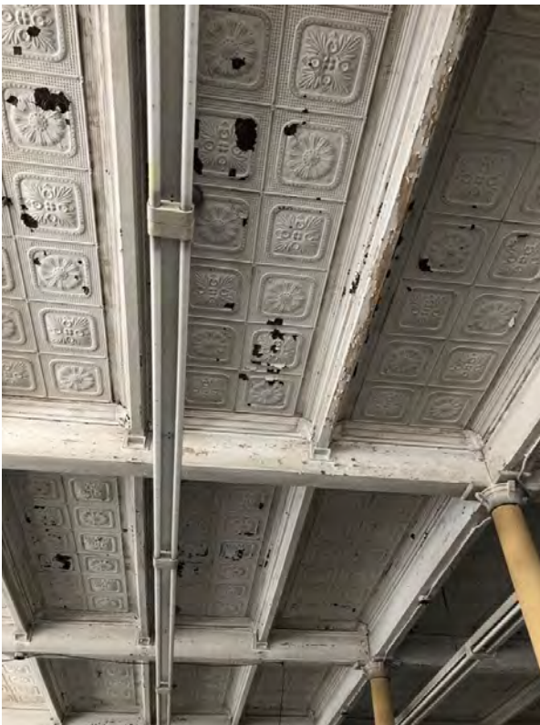
Photo 5, Ceiling detail, 1 st floor
