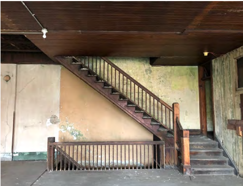
Photo 11, Stairs, 3 rd floor, looking N
