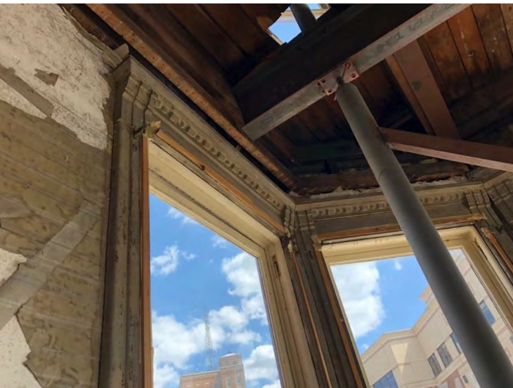
Photo 7 Turret Detail, 3 rd Floor, looking SE
