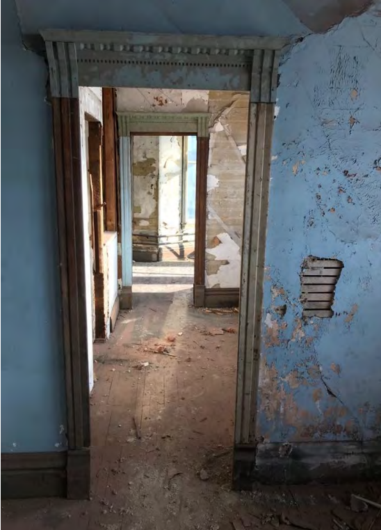
Photo 8, Doors, 2 nd floor, looking E
