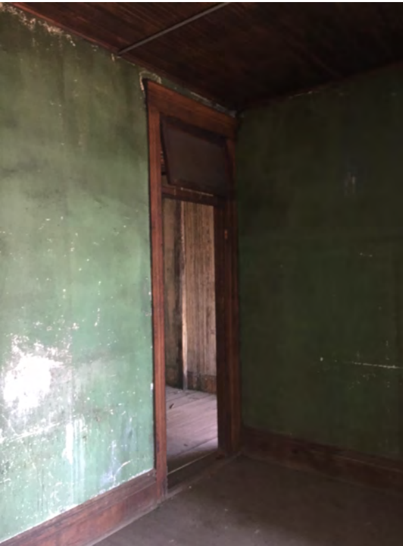
Photo 9, interior room 4 th floor, looking NE
