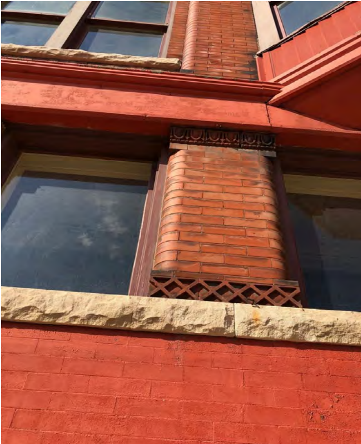
Photo 2, masonry detail on South façade, looking N
