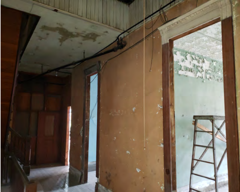
Photo 10, 2 nd floor corridor, looking SE
