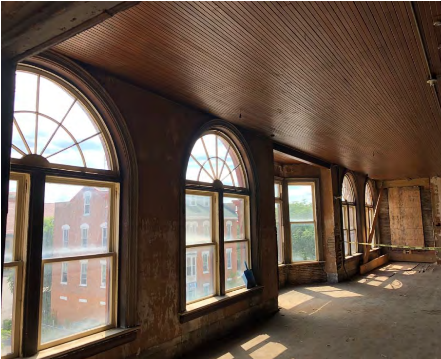
Photo 12, Bay Windows, 3 rd floor, looking SW
