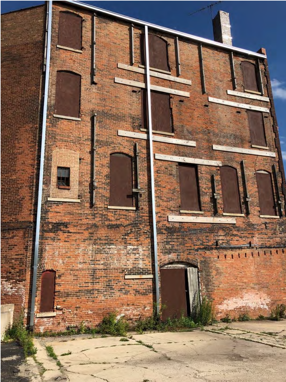
Photo 3, Rear (West) façade, looking E
