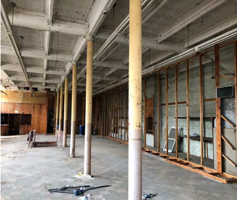
Photo 4, First floor, looking NW
