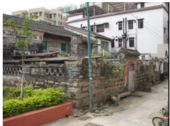
Photograph 13 Old Village House outside Wall of Tai Wai
