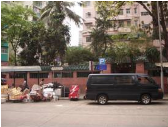
Photograph 89 Surrounding Wall of To Kwa Wan Tin Hau Temple
