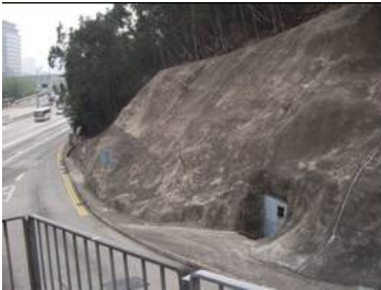
Photograph 107 Air Raid Precaution Tunnel
