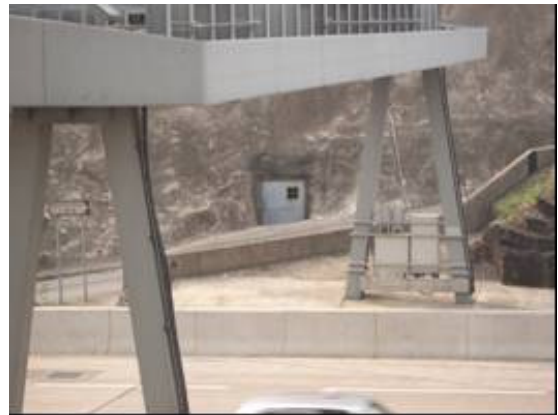
Photograph 108 Air Raid Precaution Tunnel
