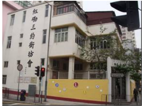
Photograph 100 Side View of Saam Yeuk Kaifong Association
