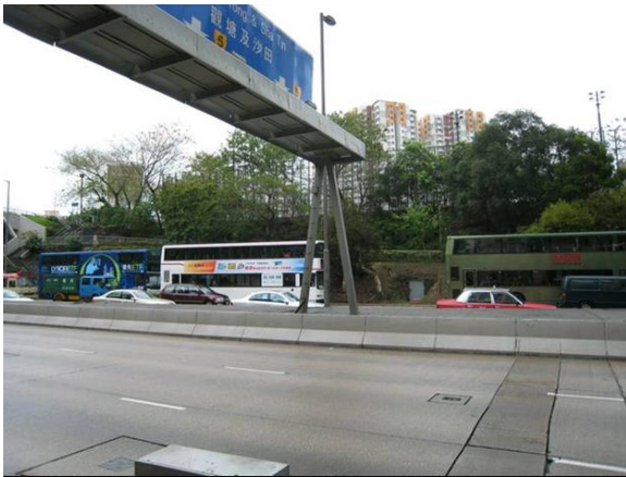
Photograph 105 Tunnel Network K4
