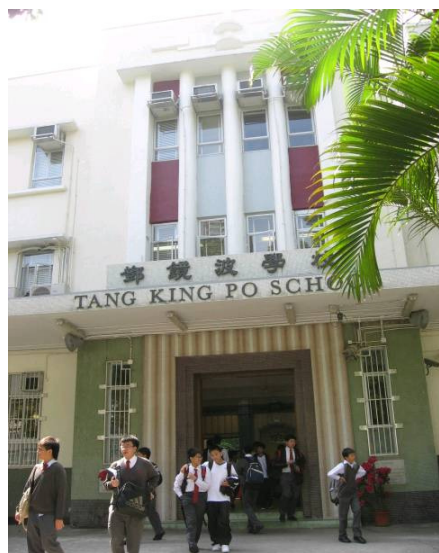
Photograph 67 Entrance of TKP School
