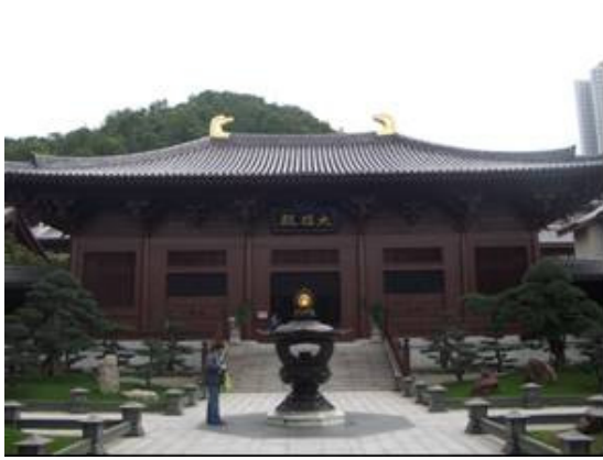
Photograph 51 Main Hall of Monastery
