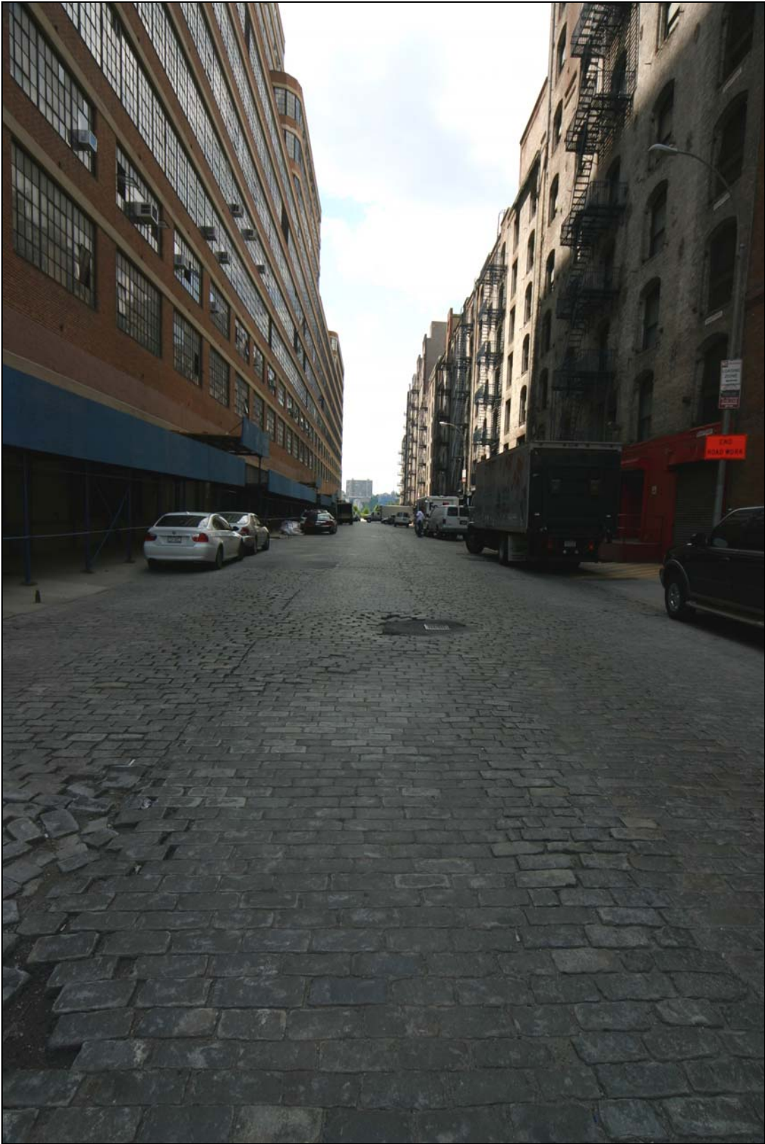
Figure 1 Granite Belgian Block Paving West 27 th Street, between Eleventh and Twelfth Avenues Photo: Christopher D. Brazee
