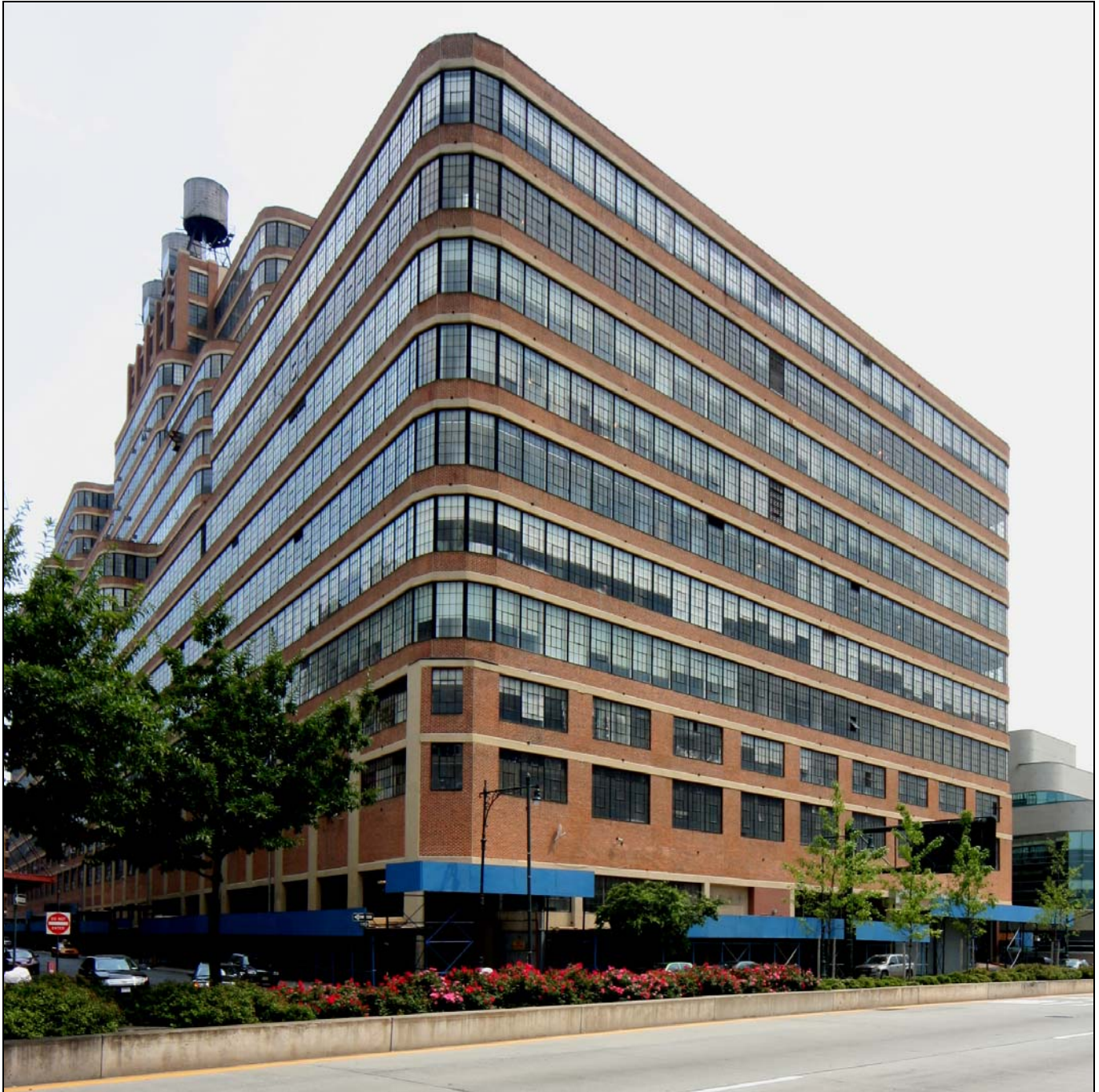
Figure 18 601 West 26 th Street Russell G. and Walter M. Cory, Yasuo Matsui, associate, 1930-31 Photo: Christopher D. Brazee
