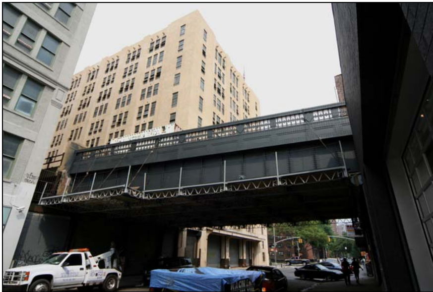
Figure 2 507-509 West 25 th Street (aka the High Line) Photo: Christopher D. Brazee
