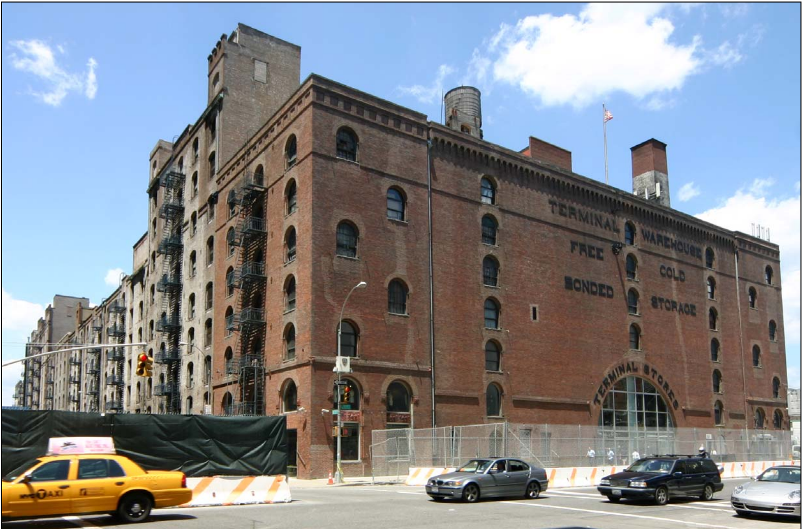
Figure 31 261 Eleventh Avenue George B. Mallory and Otto M. Beck, 1890-91, 1910-11, 1912-14 Photo: Christopher D. Brazee
