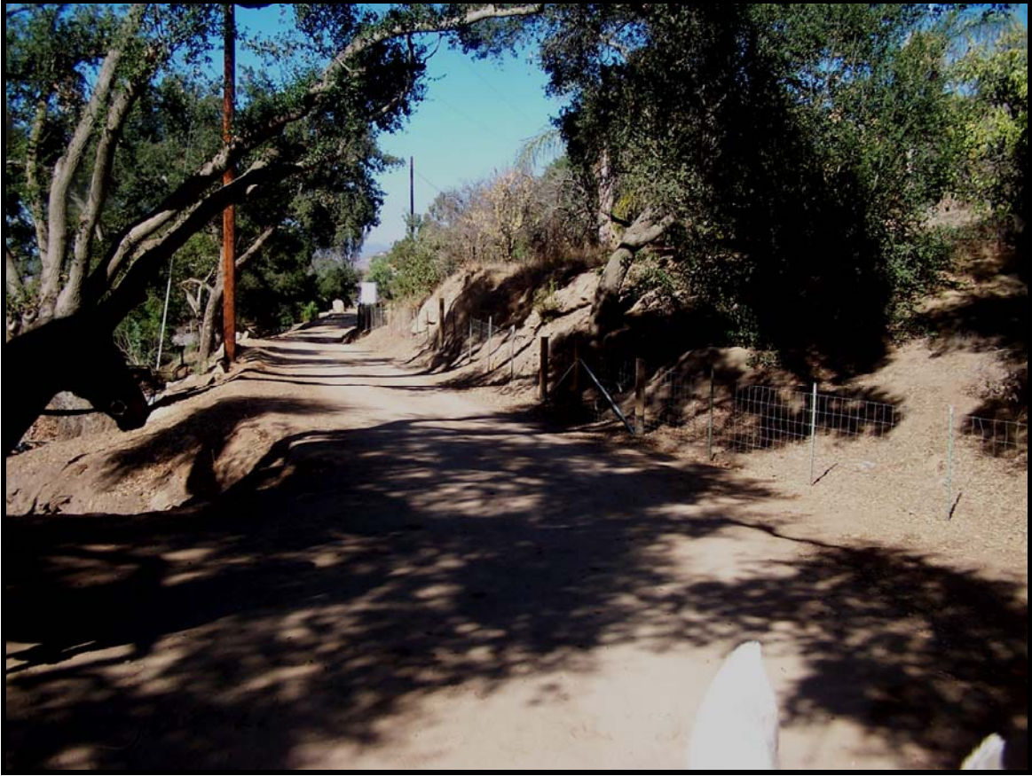
Figure 6: Old Survey Road 97 about \frac{3}{4} of a mile from the intersection with Bandy Canyon Road. Here the old road bed has not been impacted by modern grading and is closer to its original width and grade.
