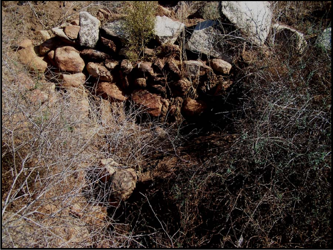
Figure 13: A second dry stacked stone retaining wall supporting the road.
