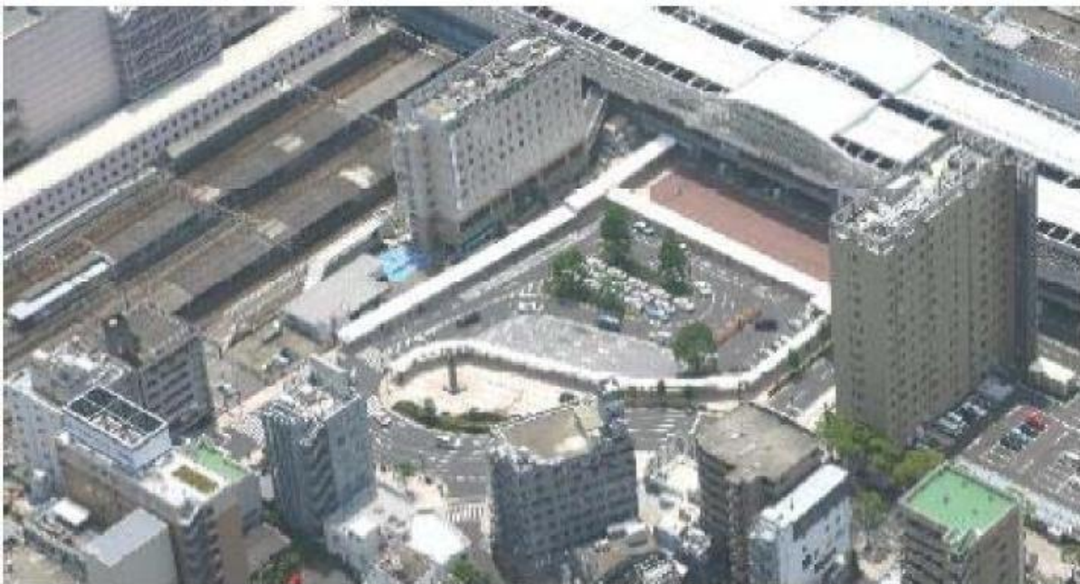
Figure 22: Station square in front of the west exit
