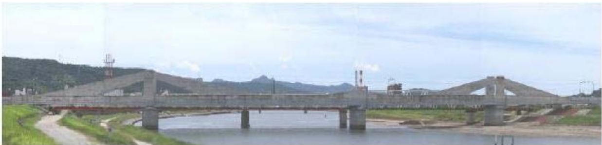
Figure 35: Sendai River Bridge
