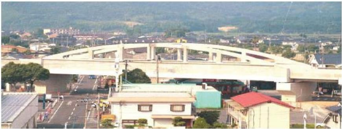
Figure 27: Harada pedestrian bridge over the Kyushu Shinkansen railway
