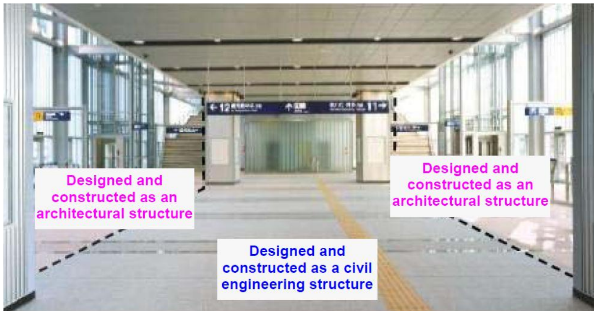
Figure 28: Structures and space inside the ticket barrier in Izumi Station
