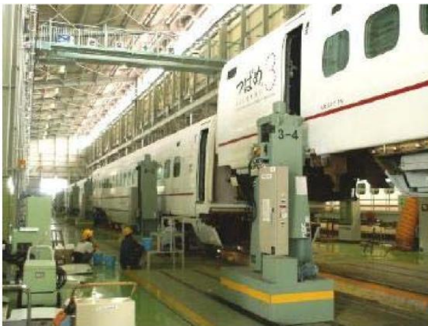
Figure 33: Car body lifting and moving equipment
