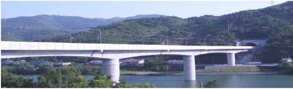
Figure 34: Kuma River Bridge
