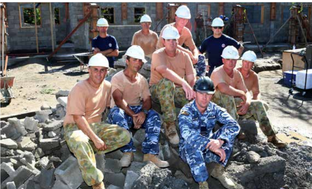
No. 65 Airfield Engineer Squadron personnel at the site of a new school house they helped build during Exercise Pacific Partnership in East Timor. Photos: SGT Pete Gammie
