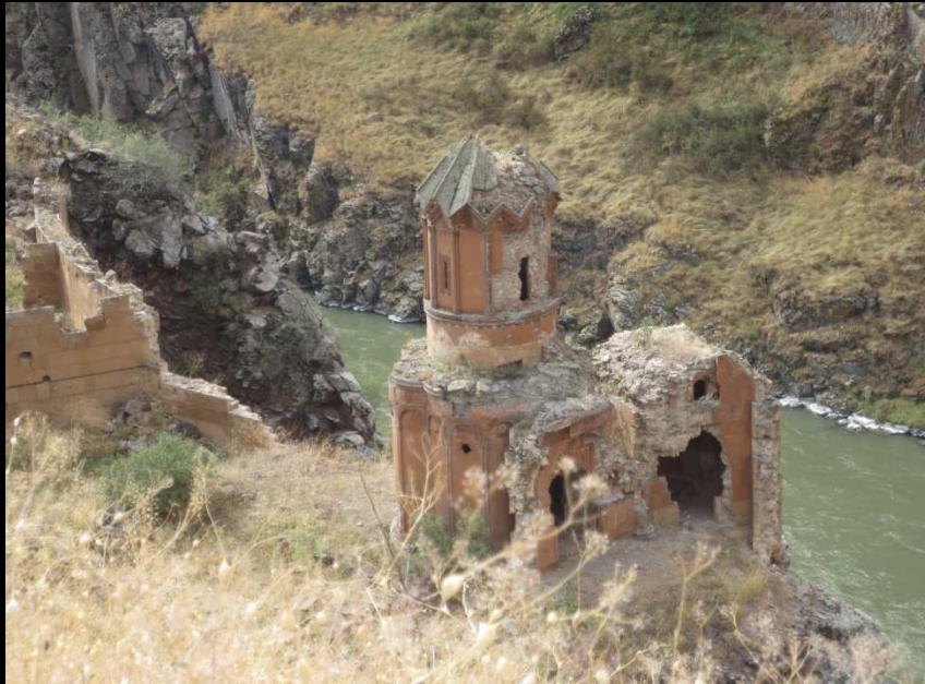
PHOTO 82: Virgins Monastery, Church, Gavit and Chapel
