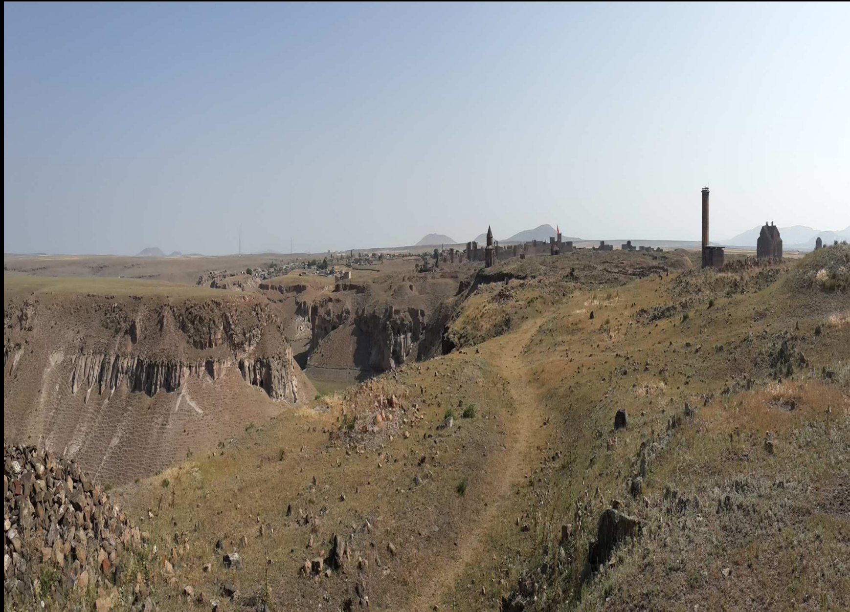
PHOTO 1: General view from south to north
