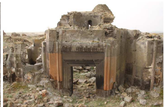
Door opening in northern façade
