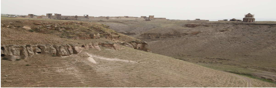
Bostanlar Creek, rock-cut structures
