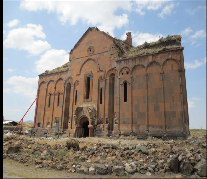
PHOTO 53: Cathedral, south façade
