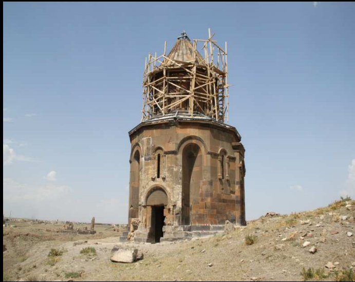
PHOTO 68: Abughamrents Church, Southeast façade
