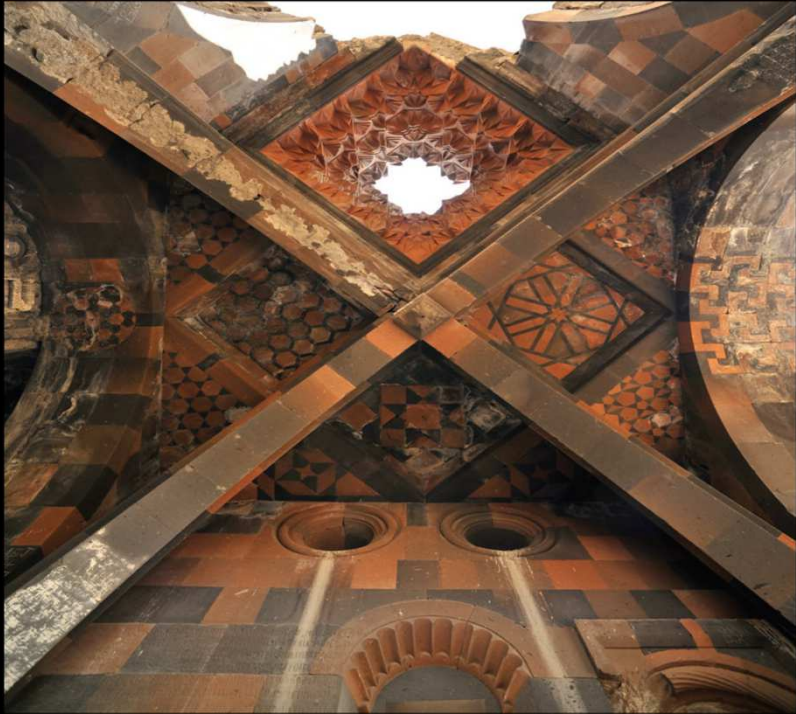
PHOTO 36: Surp Arak'elots Church, cross-ribbed vault
