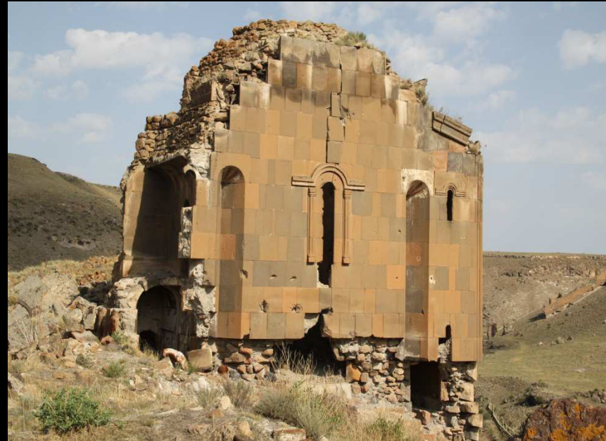
PHOTO 85: Maiden's Monastery, East facade
