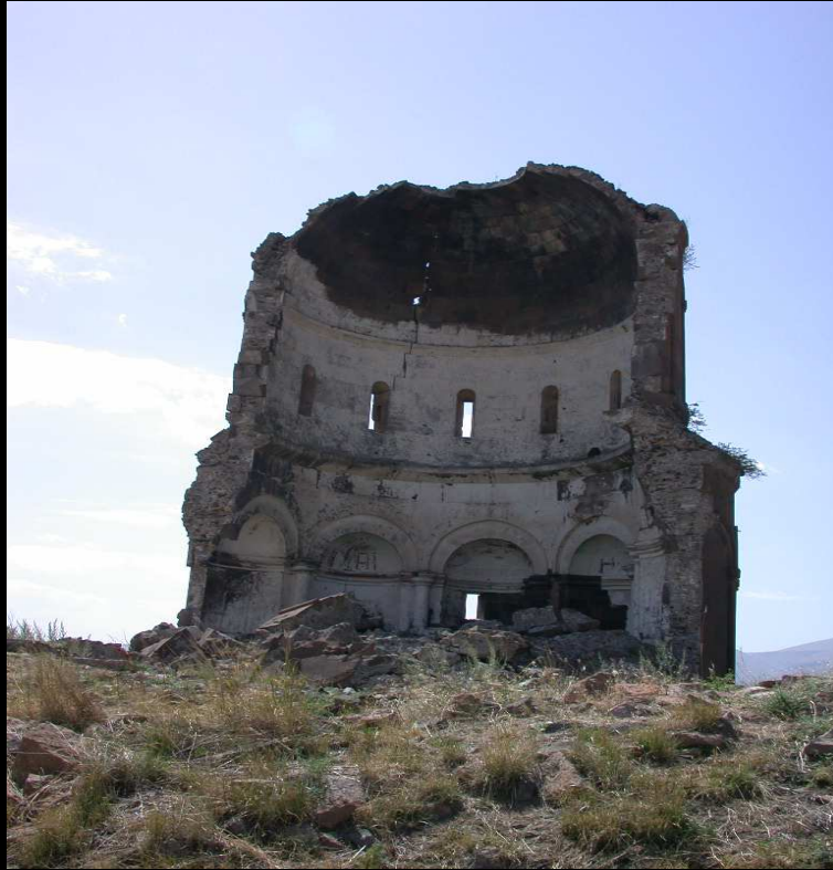
PHOTO 66: Surp Amenap'rkitch Church, West part of the church
