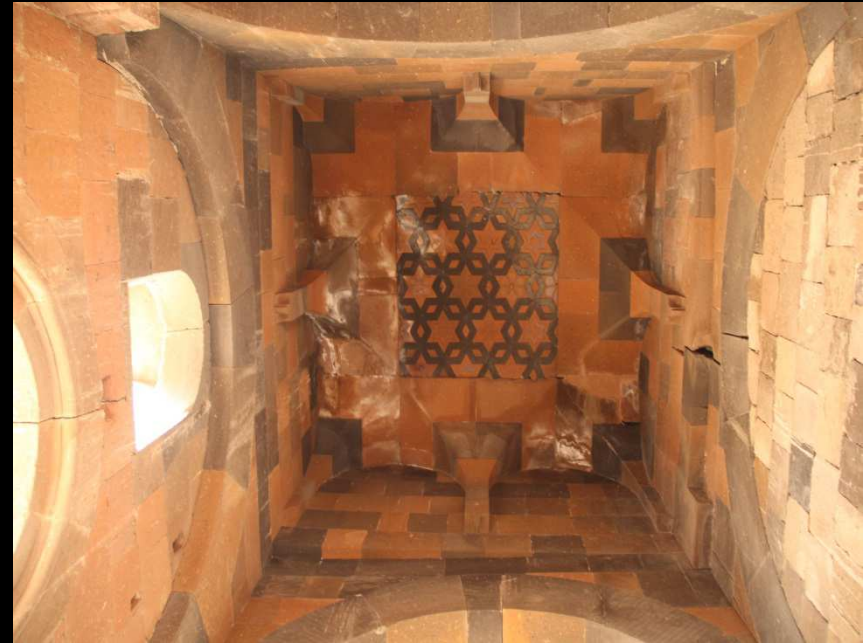
PHOTO 97: Ebu'l Manucehr Mosque, different forms of vaults
