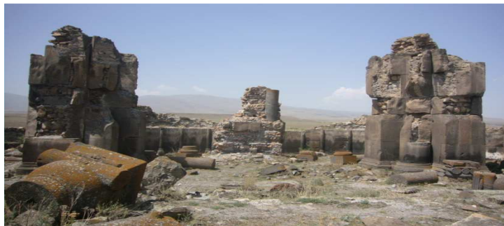
Supporting system of the church
