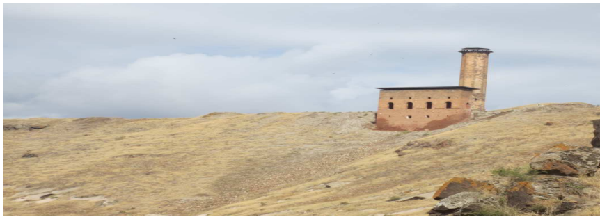
East façade of the mosque
