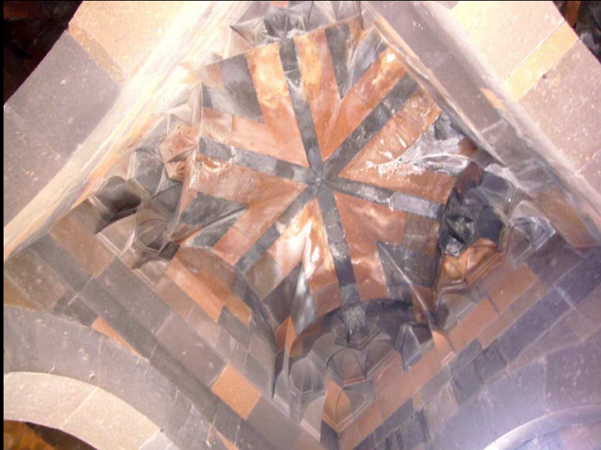
PHOTO 98: Ebu'l Manuçehr Mosque, different forms of vaults
