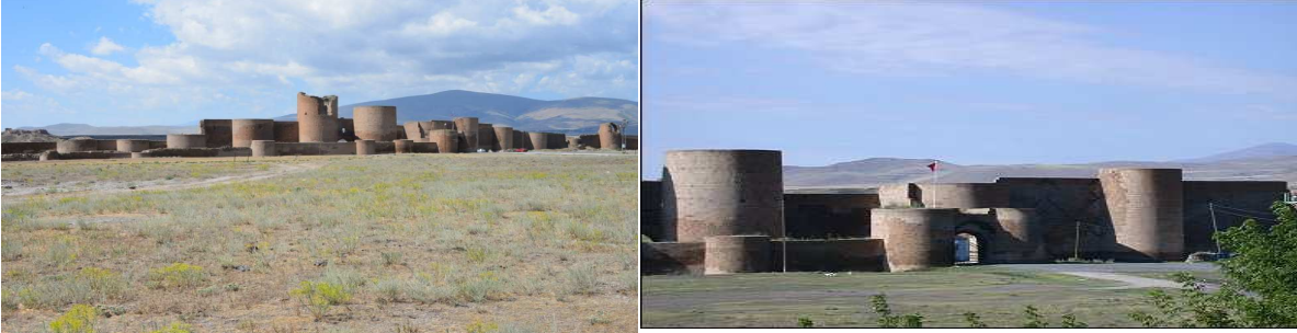
II.Smbat City Walls, view from outside
