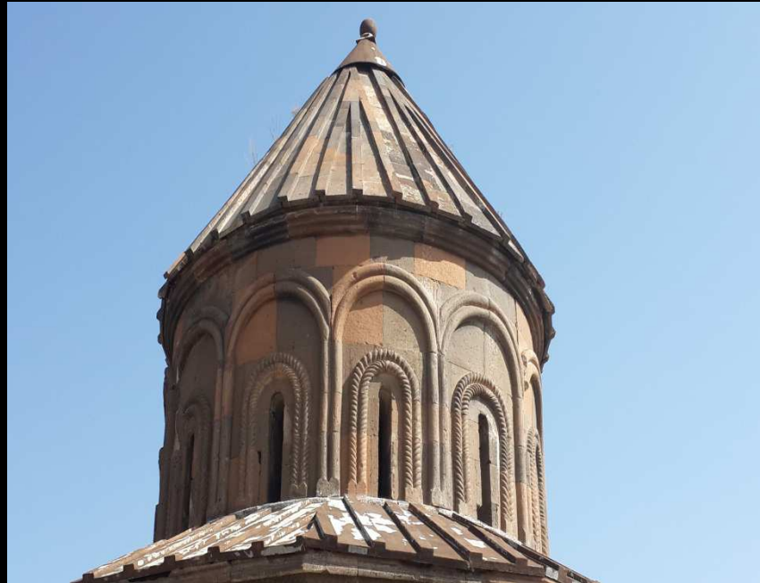
PHOTO 70: Abughamrents Church, pulley and cone
