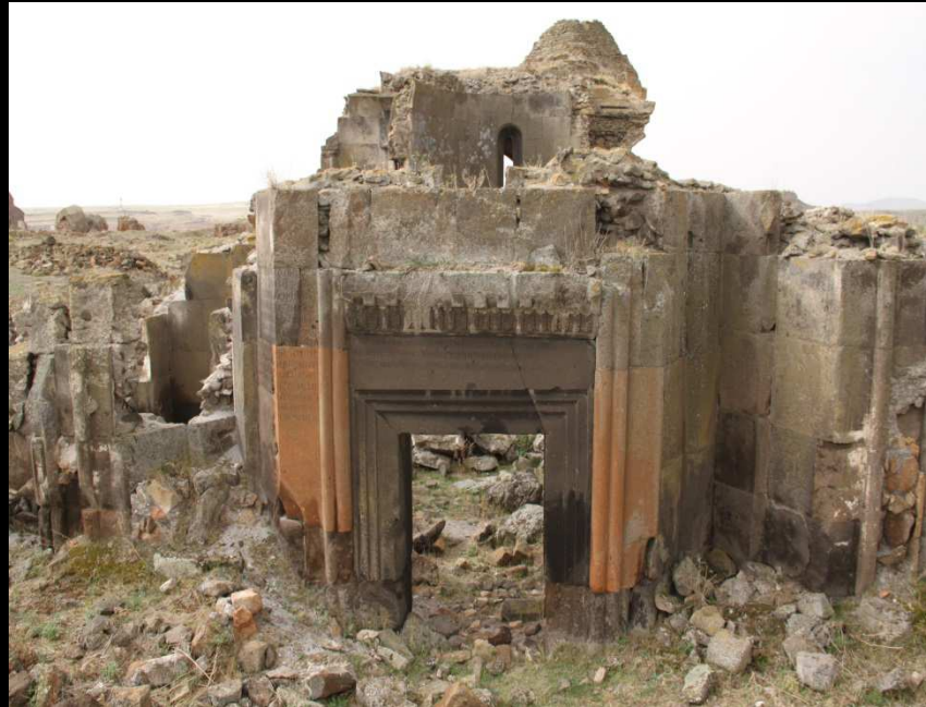
PHOTO 62: Surp Arak'elots Church, door aperture on the North facade
