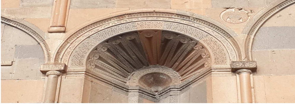
Details of figures on east façade
