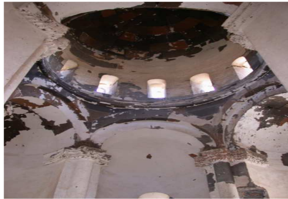
View from inside
