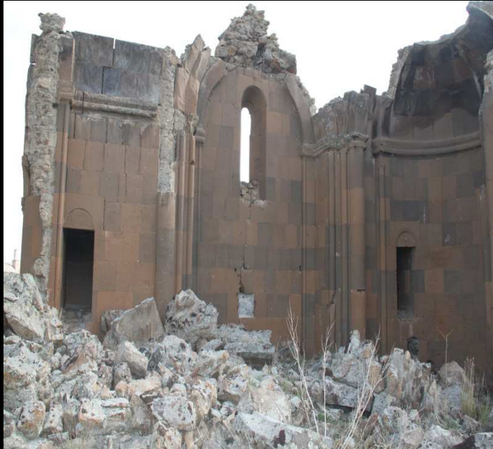
PHOTO 86: Maiden's Monastery, North wall and apse
