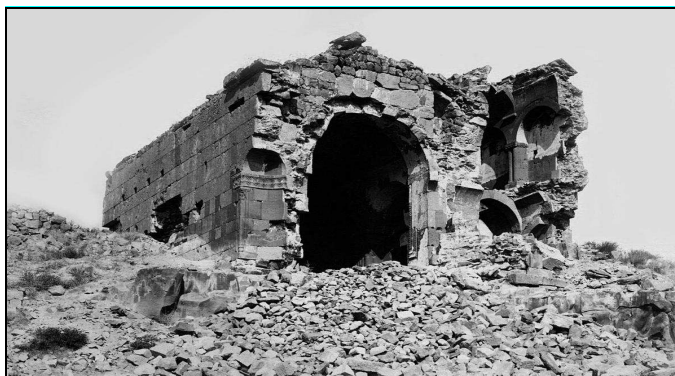
Palace Church, view from east
