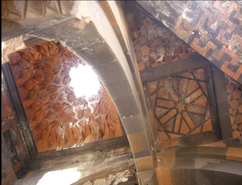
PHOTO 64: Surp Arak'elots Church, Gavit, vault system
