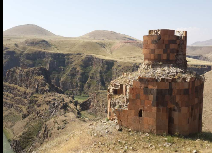
PHOTO 43: Church with six apses, view from Southeast
