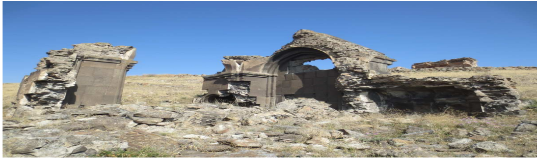
Midjnaberd Church, view from southeast
