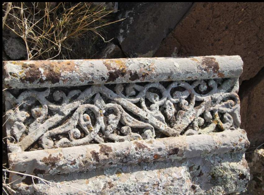
PHOTO 88: Maiden's Monastery, decorated architectural parts of structure
