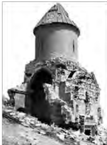
Midjnaberd Church, southeast view (Karapetian, 2011)
