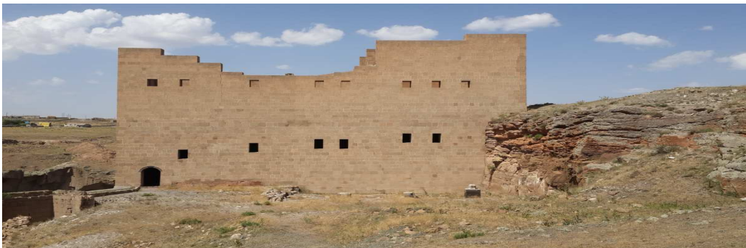
South façade, entrance to ground floor
