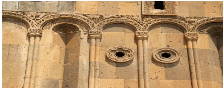
Decoration detail on south façade
