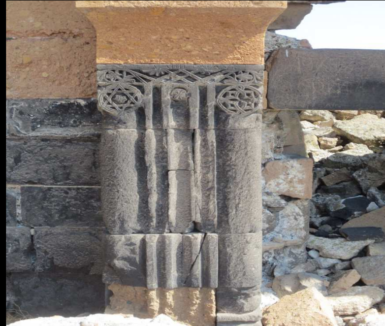
PHOTO 41: Palace Church, plaster on the North wall
