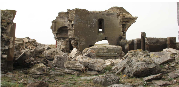
Surp Arak'elots Church, view from north
