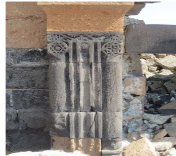
Plaster on northern wall
