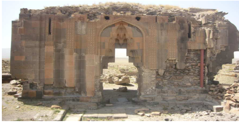
Gavit, east façade
