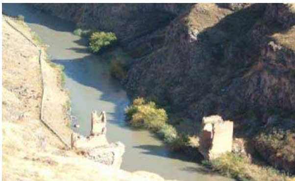
Figure 14: Silk Road Bridge on the Arpacay River Bridge ( www.karskulturturizm.gov.tr )
