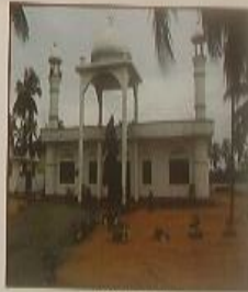
The Mosque during construction
