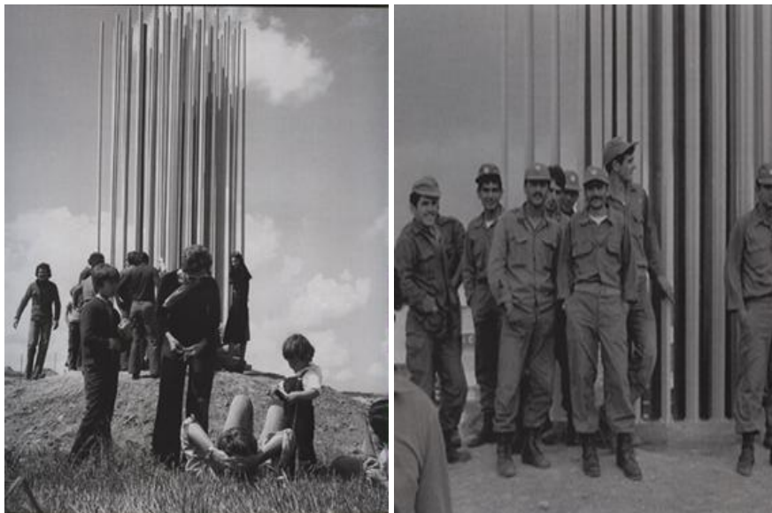
Figures 144, 145: Installing the Rainbow , 1975.
