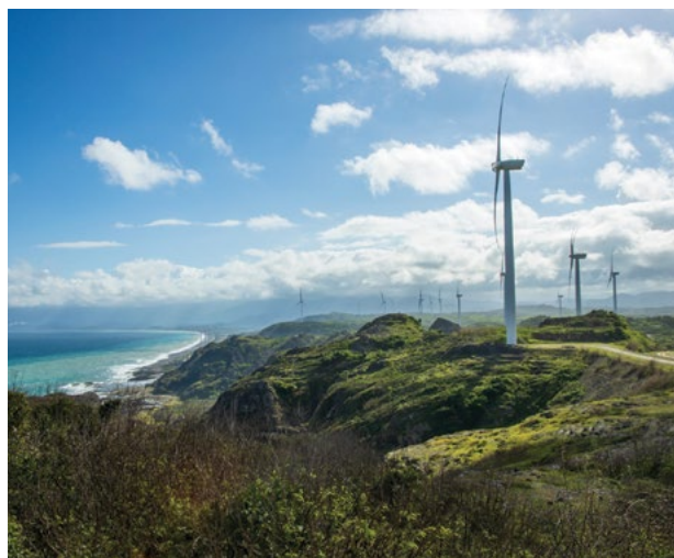
Ilocos Norte wind farm
