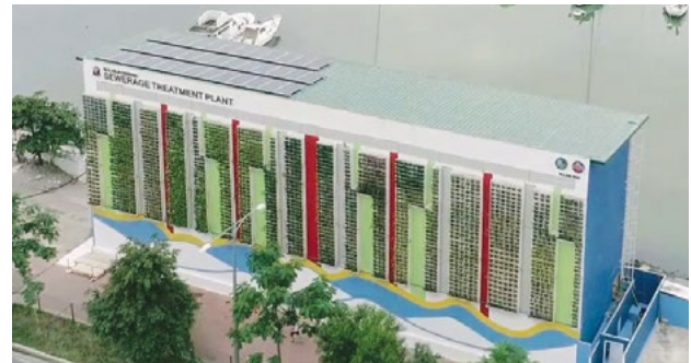
In July 2020, the DENR unveiled the country’s first solar-powered sewage treatment plant that can treat 500,000 liters/day of domestic wastewater from major drainage outfalls along Manila Bay.
