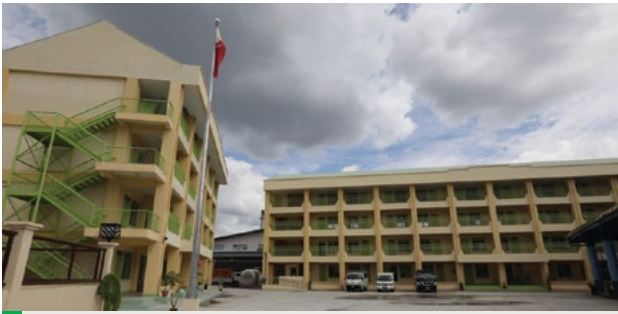
Two (2) newly constructed four-storey buildings with 24 total classrooms in Lawang Bato National High School, Valenzuela City.
