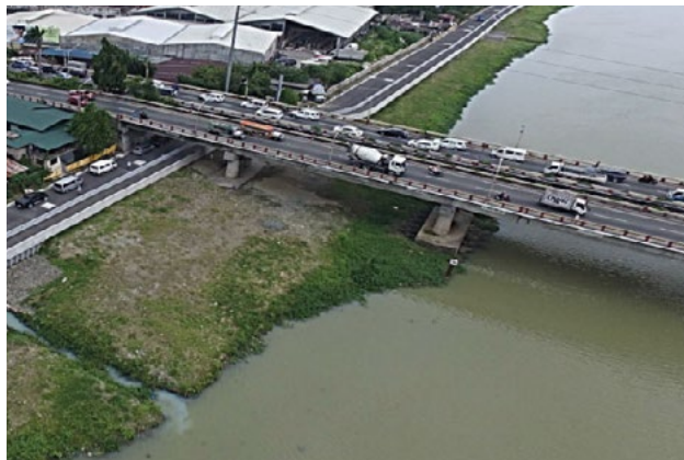
The Pasig-Marikina River Channel Improvement Project Phase III, which involves channel improvement works at the remaining sections of Pasig River and priority critical sections of Lower Marikina River, was completed in July 2020.
