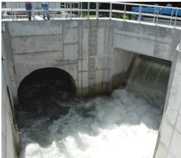
Angat Water Transmission Improvement Project - Tunnel No. 4
