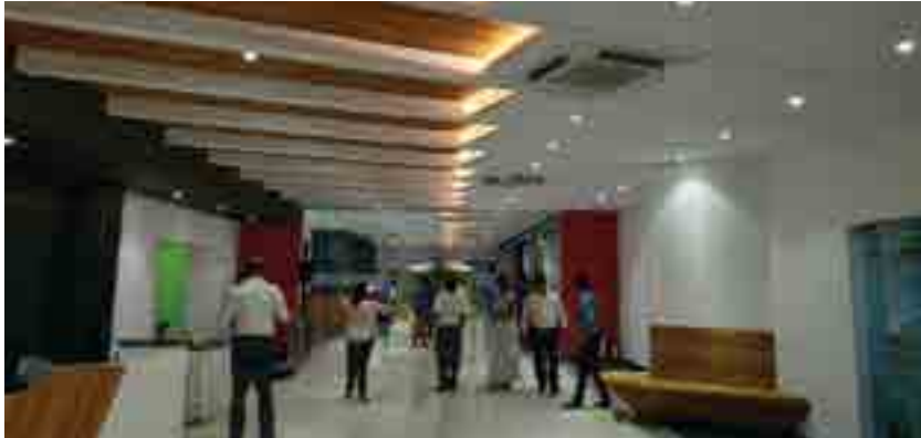
Renovation of Head Office Building
