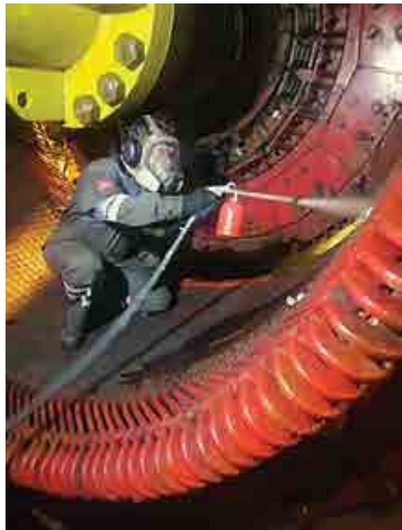
Stator winding cleaning of Generator No.04
