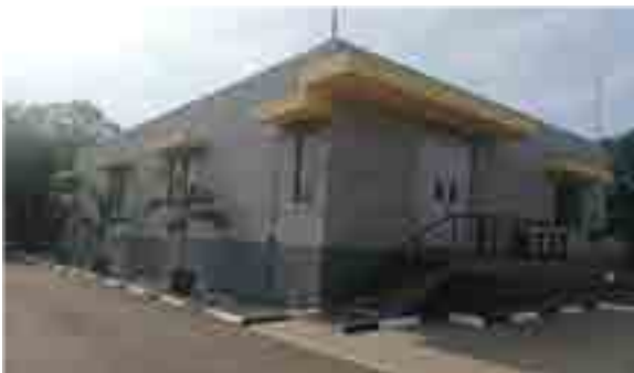
Kelanitissa 33kV GIS substation
