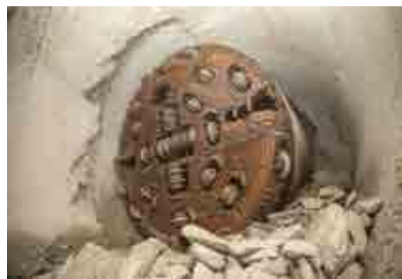
Main Tunnel Breakthrough
