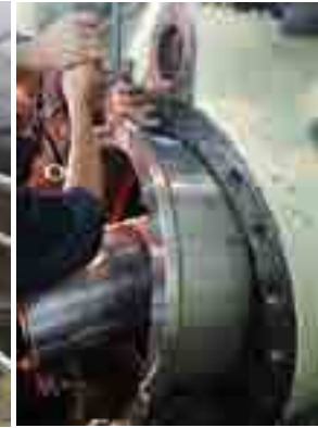
Insertion of Trunnion Bearing
