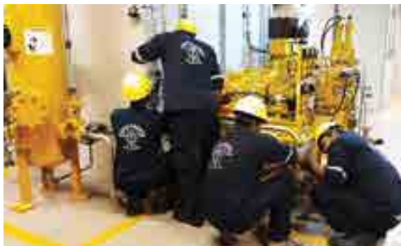
Annual maintenance of U-2 machine- Kukuleganga power plant
