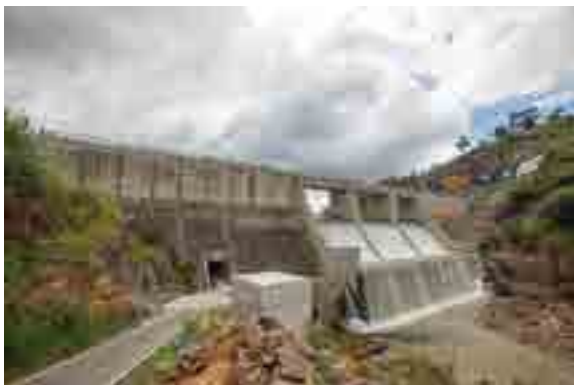
Spilling of Puhulpola Dam
