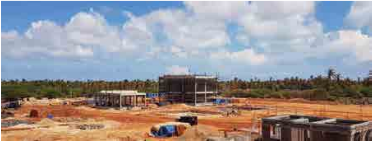
Construction works at Nadukuda GSS 220kV switchyard
