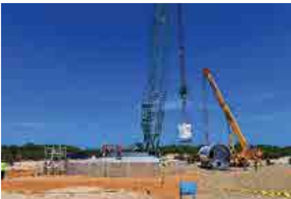
Installation works in progress - MWPP
