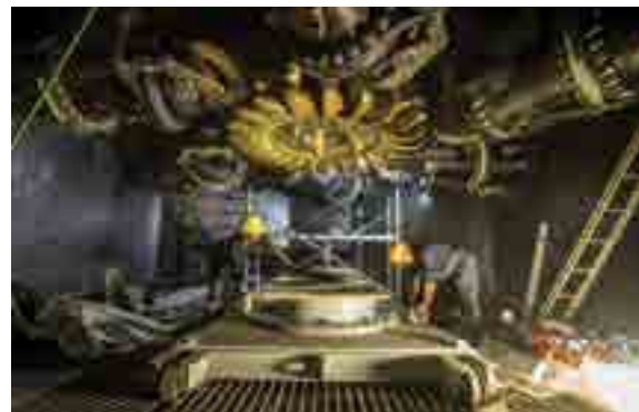
Installation of Turbine (Unit1)
