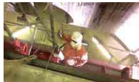
Sand Blasting and Painting of Intake Gate, Draft Tube Gates and Surge Chamber Gate at Kotmale Power Plant.
