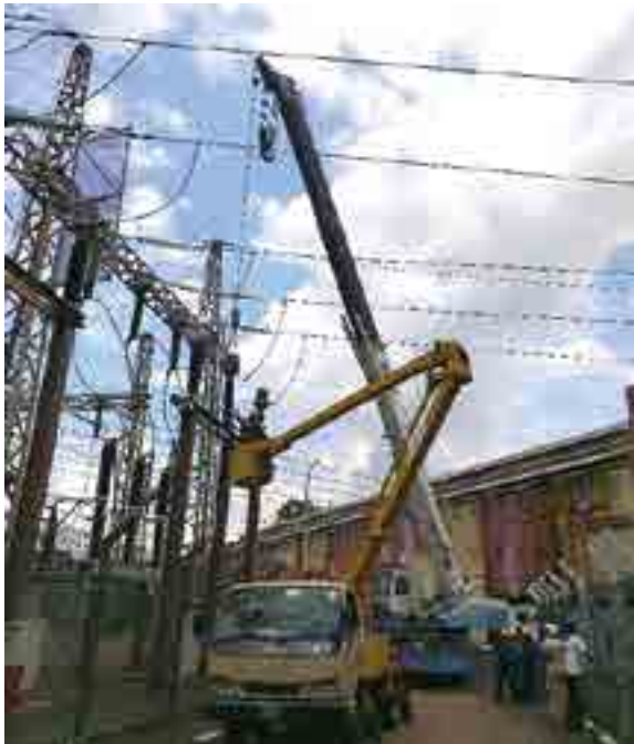
CT Replacement of Switch Yard
