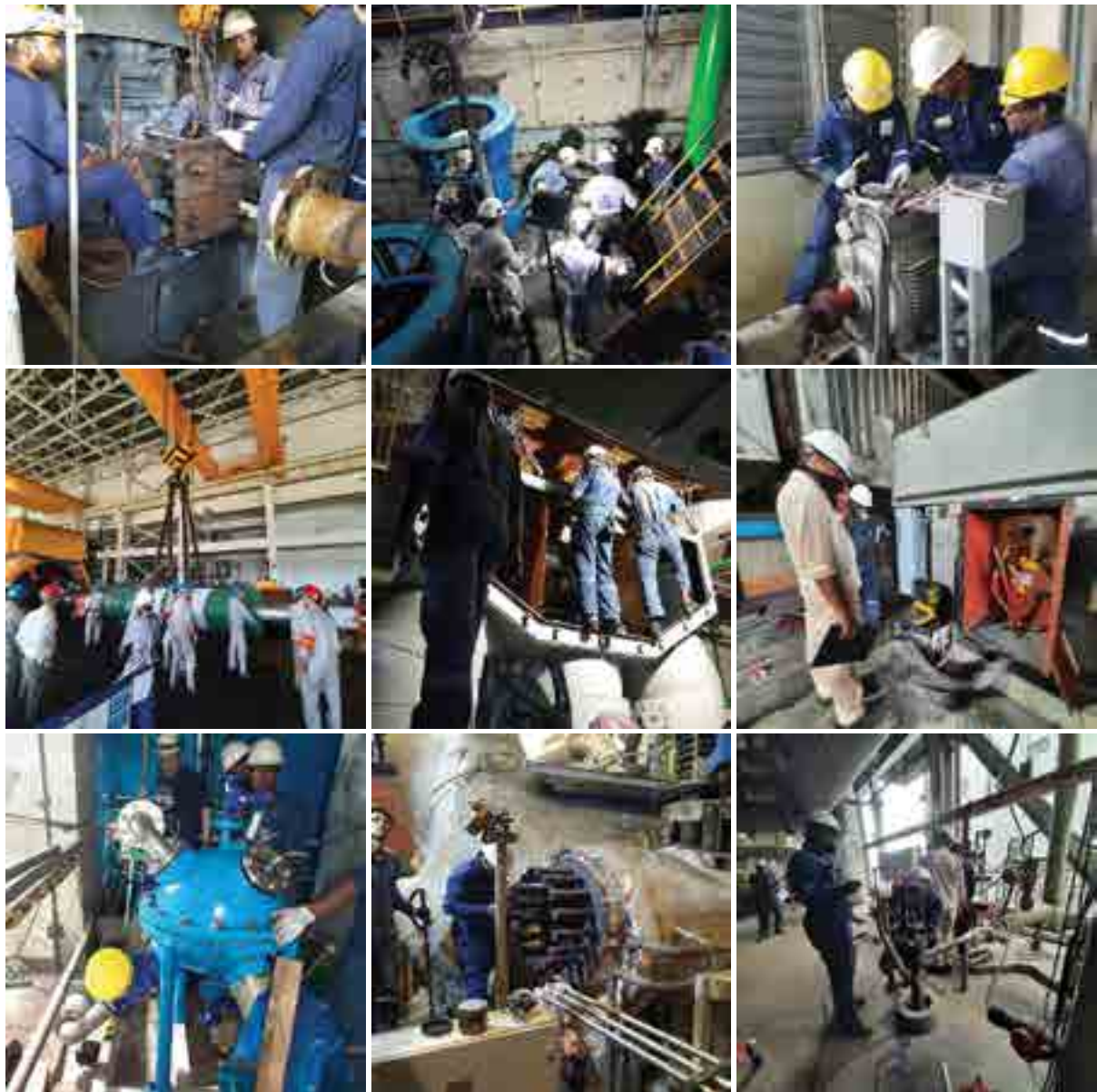
Unit 01 Overhaul- Lakvijaya Power Plant
