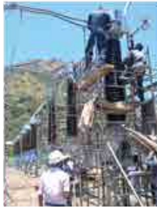
Installation in progress
