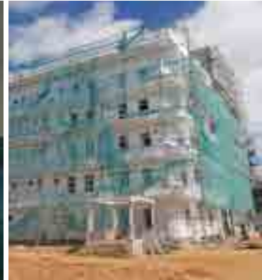
Construction of DGM(NCP) Office in Anuradhapura
