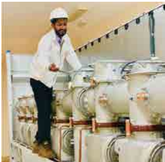
Figure Tr.9: Commissioning of 33kV GIS at Maliboda GS
