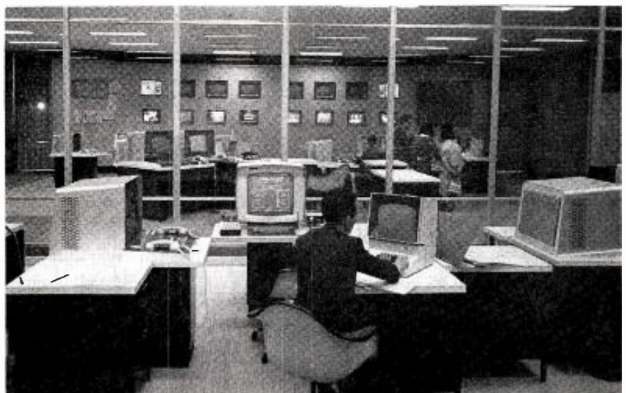
Shown above is Japan Broadcasting Corp.'s (NHK) broadcast control center which can give program managers
