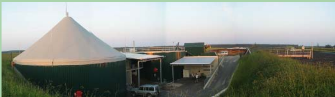
Biogas plant with digester 1, digester 2 and final storage of the digestate (Photo: Resch)
