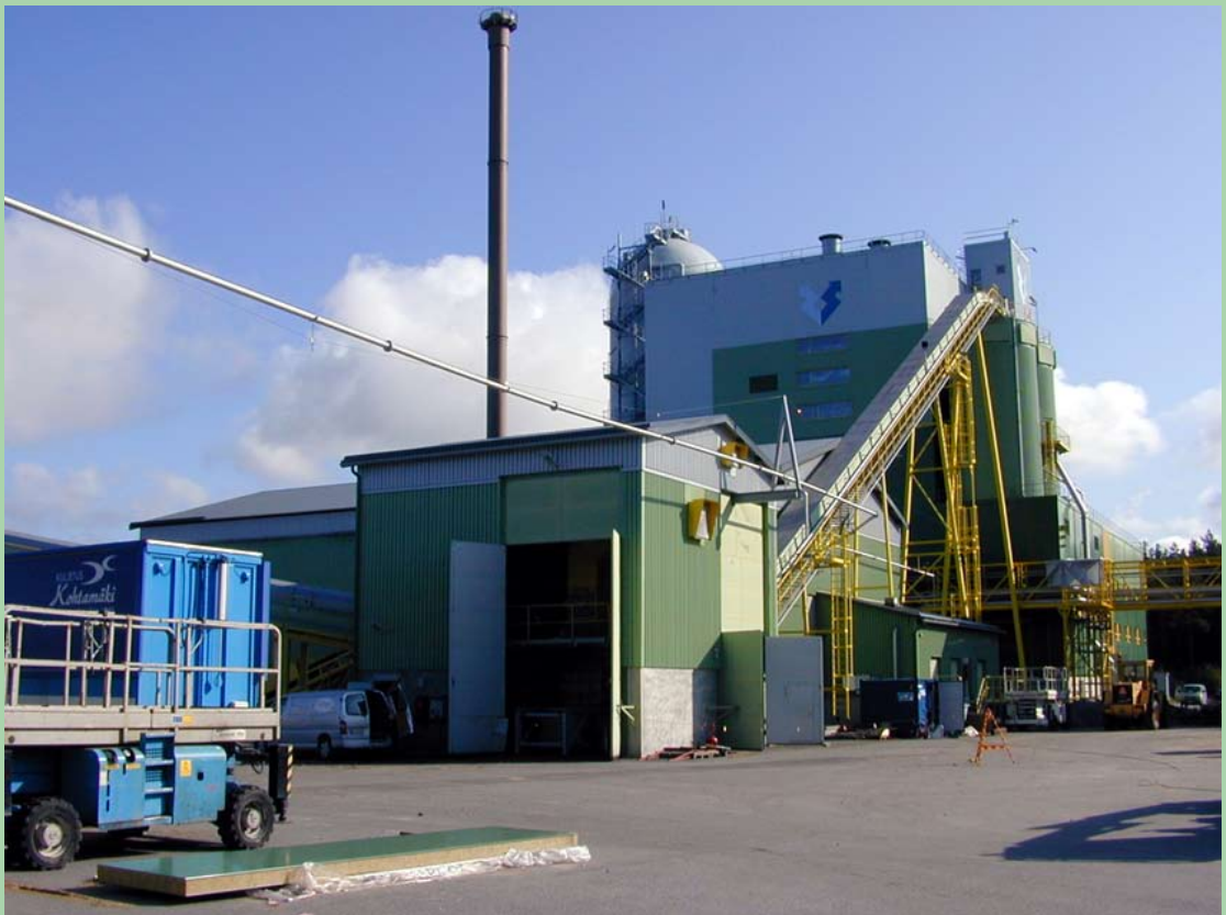
Power plant of Kokkolan Voima Ltd. Reed canary grass chop is transported pneumatically to the boiler via the pipeline on the left. (Photo: Timo Lötjönen, MTT).
