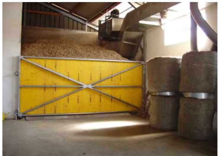
In the center box for drying wood chips; on the right - facility for drying hay. (photo: IEA Tulln, Gabauer)
