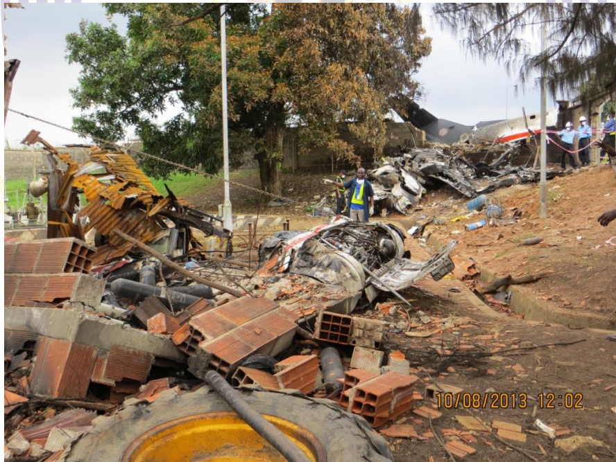
Figure 9: The Aircraft Engine and Generator Room destroyed by post impact fire
