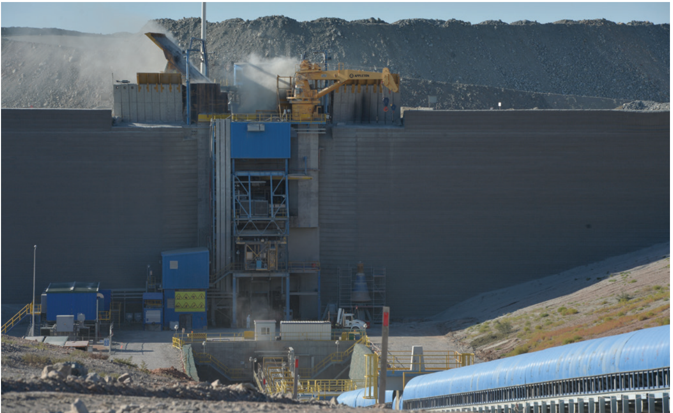
The primary cone crusher located at the open pit has 525 tonnes capacity and can crush up to 6,086 tonnes of material in an hour. The crusher reduces the ore in size to around 200 millimetres.
