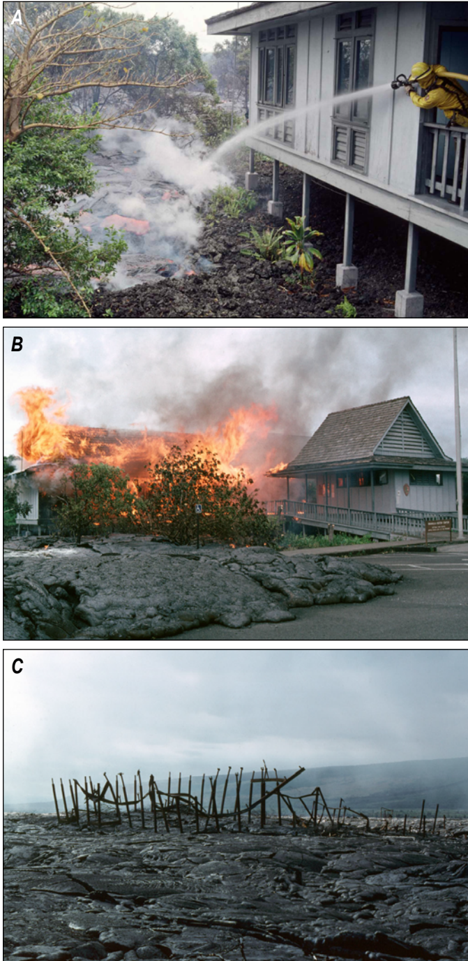
Figure 6. Photographs of the National Park Service Waha'ula Visitor Center near the coast on Kilauea Volcano in 1989 and of efforts to protect it from approaching lava. A , Fire hose delivers water to cool approaching pāhoehoe flows (June 22, 1989). B , Visitor Center engulfed in flames later that day after being ignited by hot lava. C , Steel girders, twisted by inflating lava flows and later buried, are all that remain of the Visitor Center after it burned (October 12, 1989). U.S. Geological Survey photographs by Jim Griggs.
