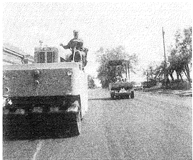
Paving Main Street in Oak Lake.
