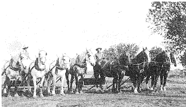
Trans-Canada Highway "Trimmers". D. A. Taylor, Contractor 1934.
