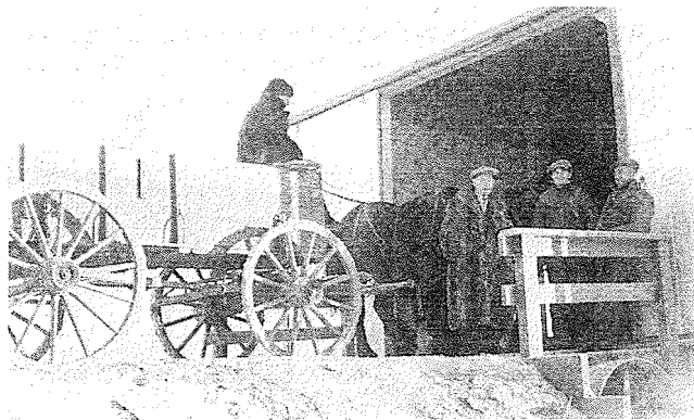
Nelson Banister delivering grain to Wilfred Gordon at new Ogilvie Elevator.
