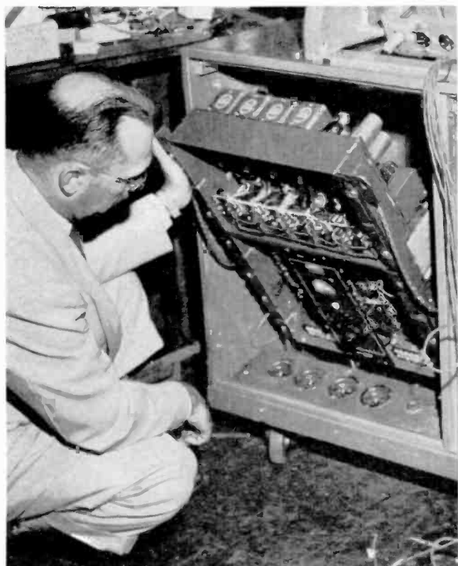
The amplifiers are pivoted for instant servicing or adjustment. Here Altec engineer Martin Bender shows how the unit swings down.
