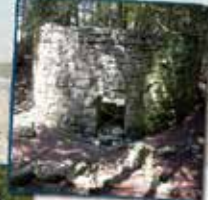
Limestone chunks buried in simple pits produced 'quartz lime'. This powder was used as mortar to hold stone and brick, and as whitewash to seal fence walls on pasture and orchard tree trunks.
