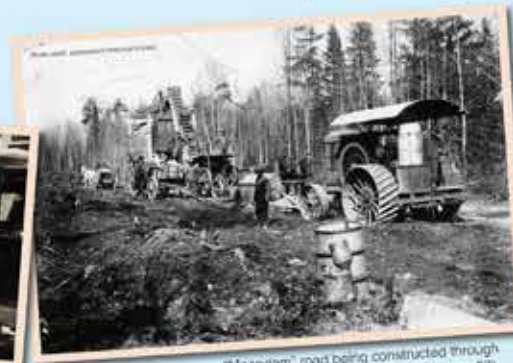
"Macadam" road being constructed through Jacksonport circa 1916 (now Highway 57).
