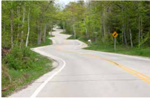
This curvy section of Highway 42 in Liberty Grove was designed by Jens Jensen, a prominent landscape architect who established The Clearing in Ellison Bay. His idea was to slow down traffic so visitors could better appreciate the scenery.
