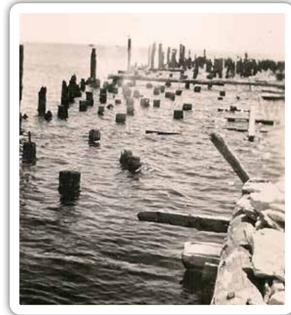
In 1938, ice damaged the Jacksonport piers beyond repair.
