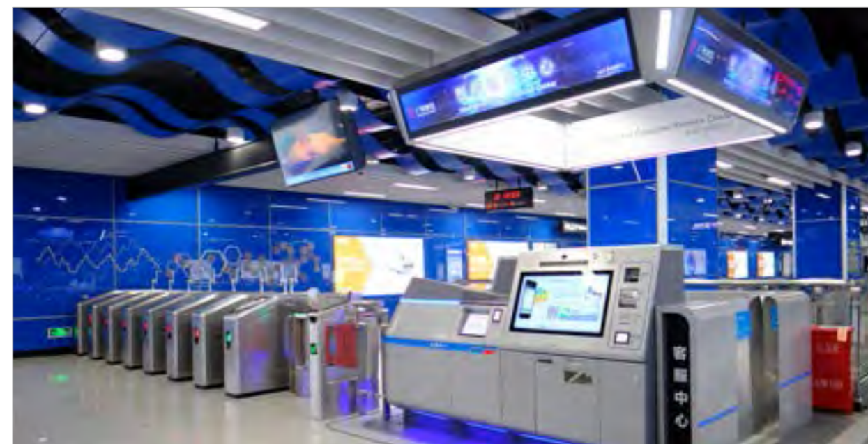
9月9日，智慧地铁示范站在地铁三号线广州塔站和二十一号线天河智慧城站正式上线，并发布轨交智慧操作系统——穗腾OS1.0。On September 9th, the intelligent metro demonstration station was officially launched at Tianhe Smart City Station of Line 21 and Canton Tower Station of Line 3. The intelligent operation system for rail transit, Suiteng OS1.0, was also released on the same day.
