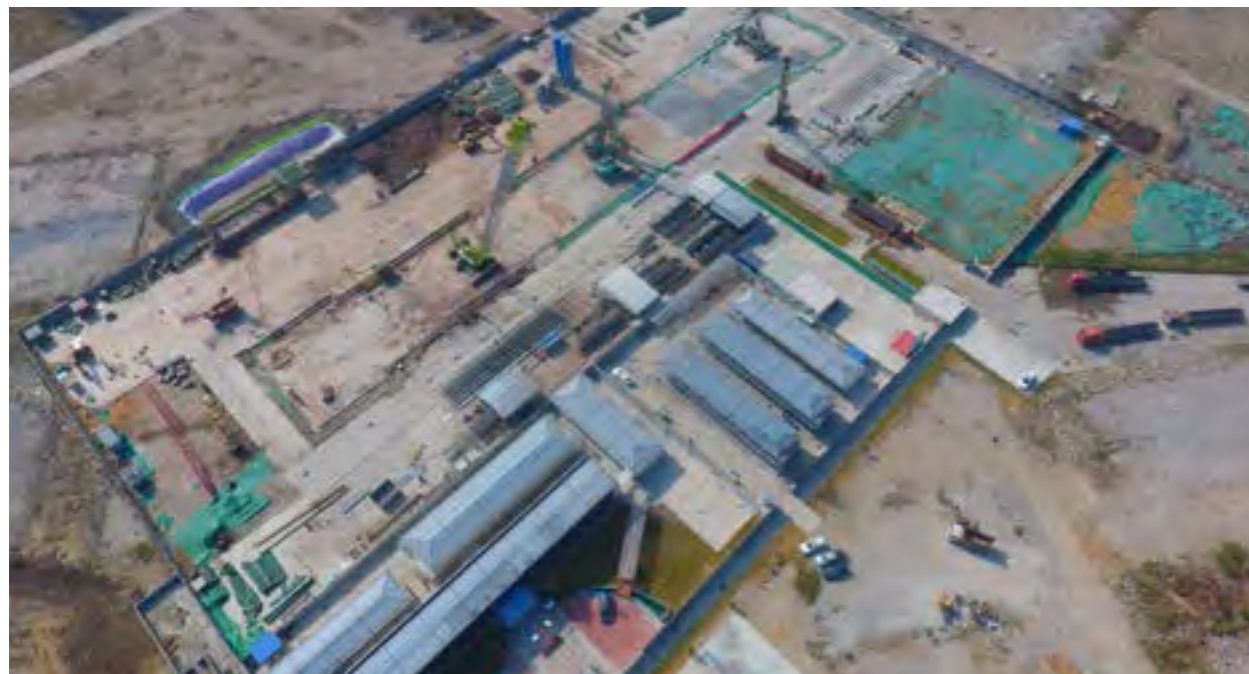
七号线洪圣沙站 Hongshengsha Station of Line 7
