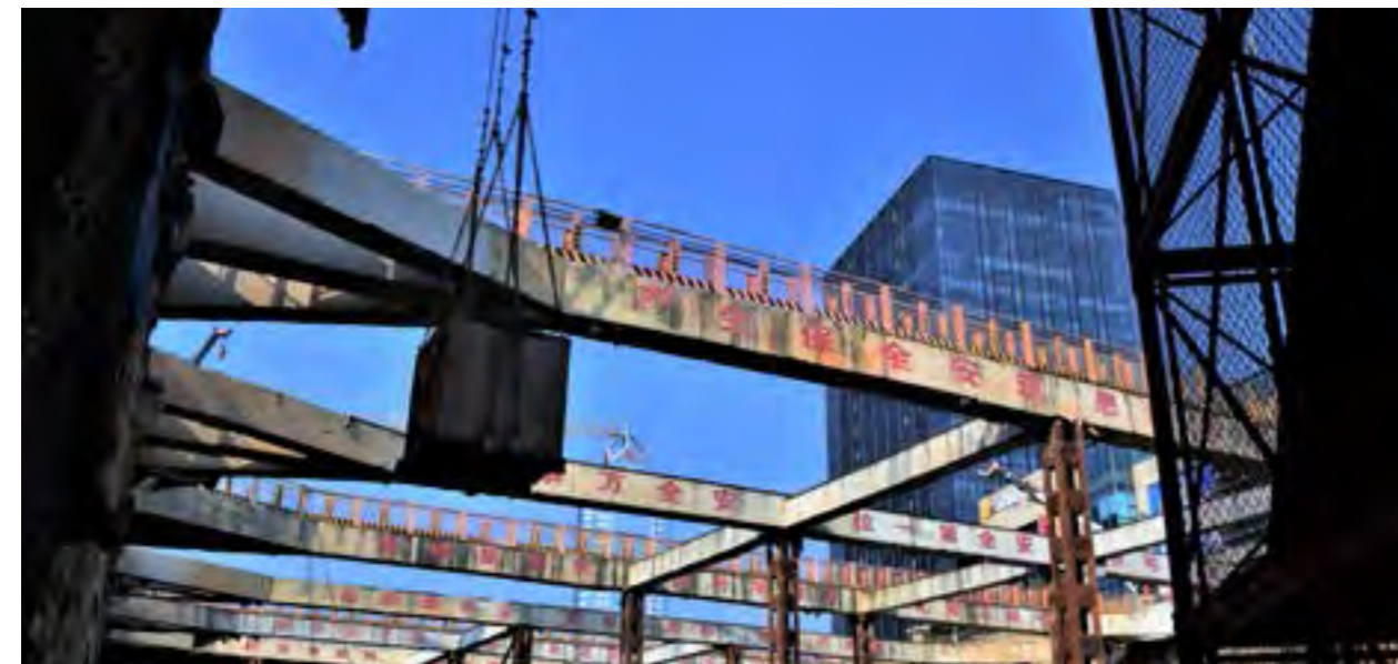
十八号线番禺广场站 Panyu Square Station of Line 18
