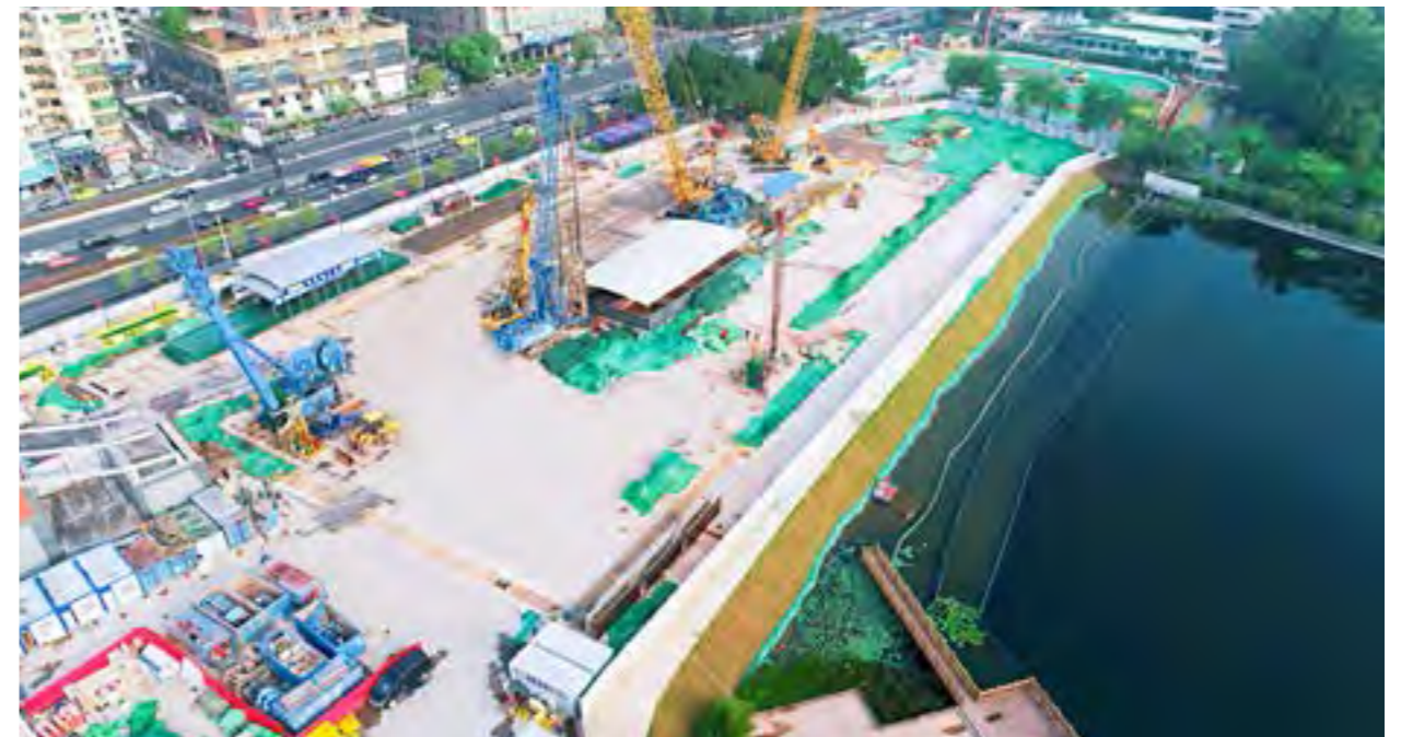
十号线东湖站 Donghu Station of Line 10
