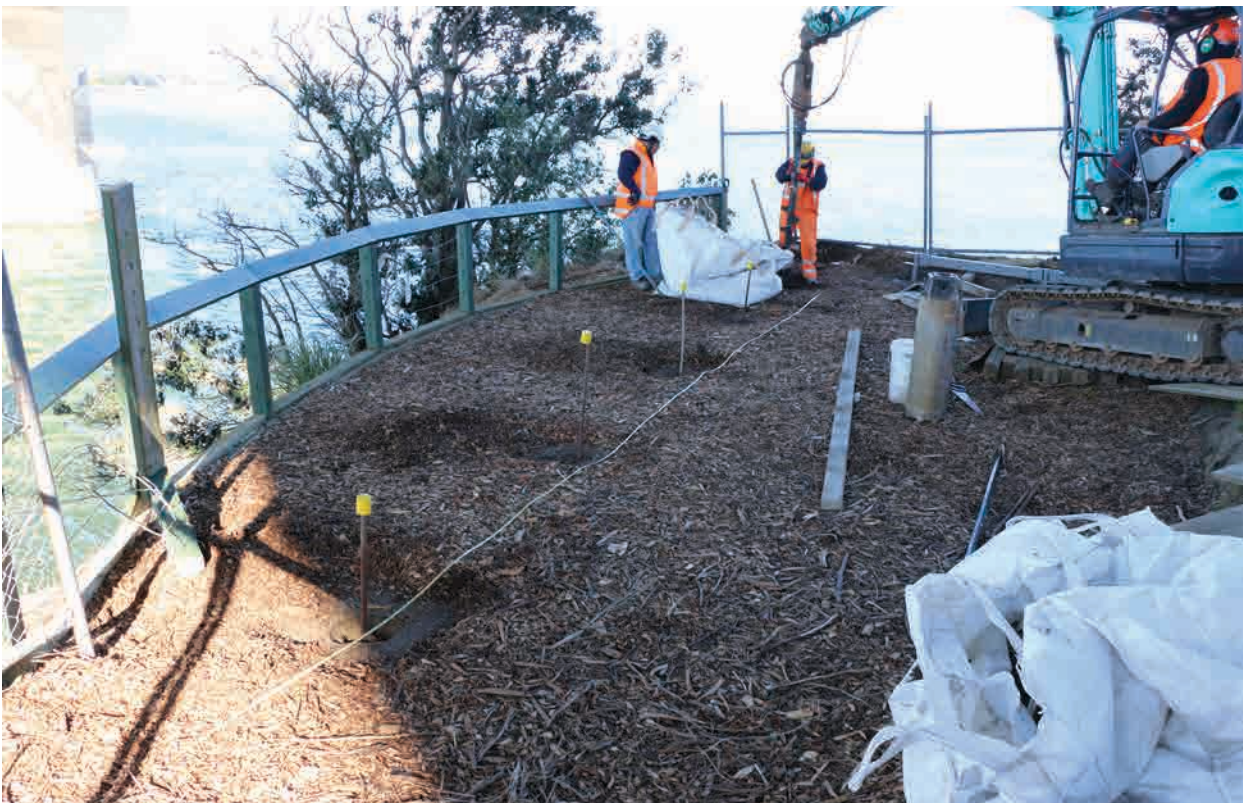
Figure 15. View south of new fence post footings being augured.
