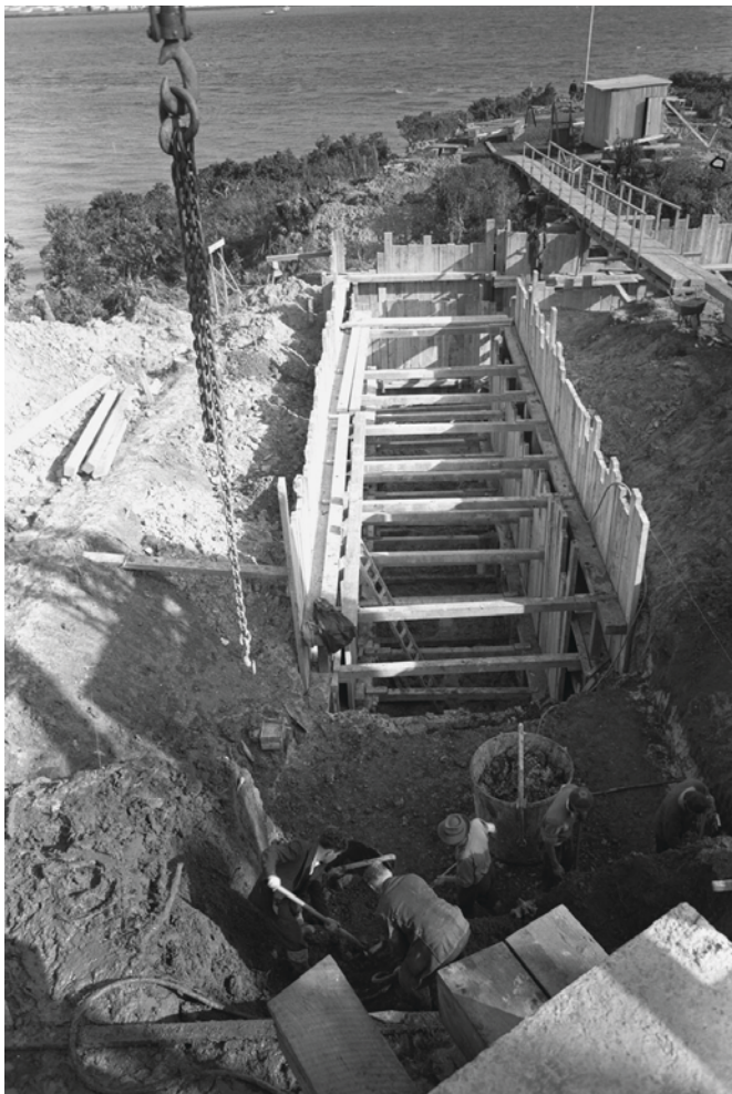
Figure 8 (above). Photo probably dated to 1957 showing the installation of a tramway along the western side of the pa. Note the pier which is being used for support, along with the stays which can be seen presumably attached to anchors to the left of frame. Sir George Grey Special Collections, Auckland Library 459-15.
