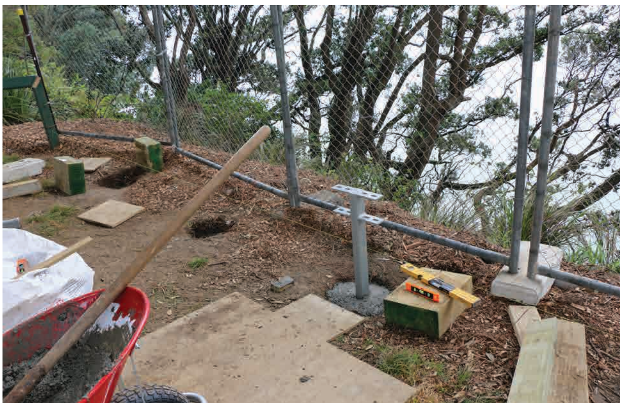
Figure 16. New fence post in place.
