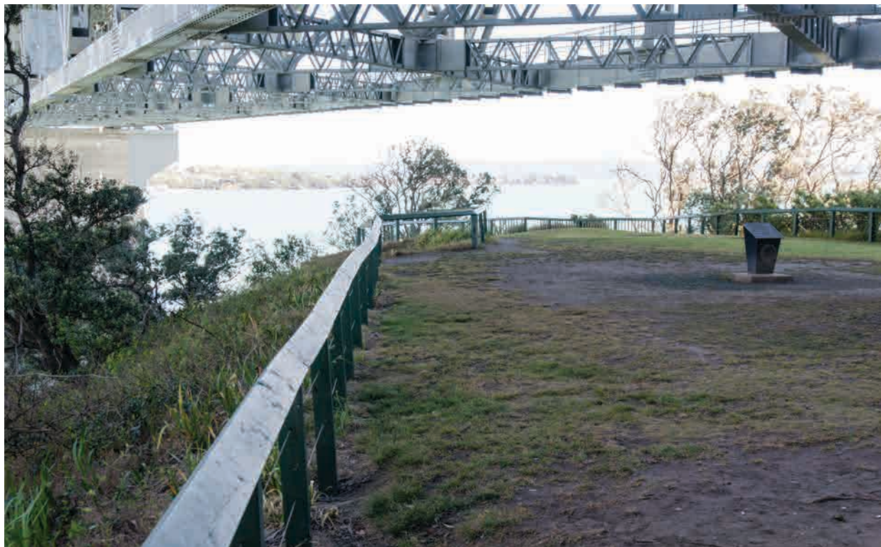
Figure 11. Previous perimeter fence.
