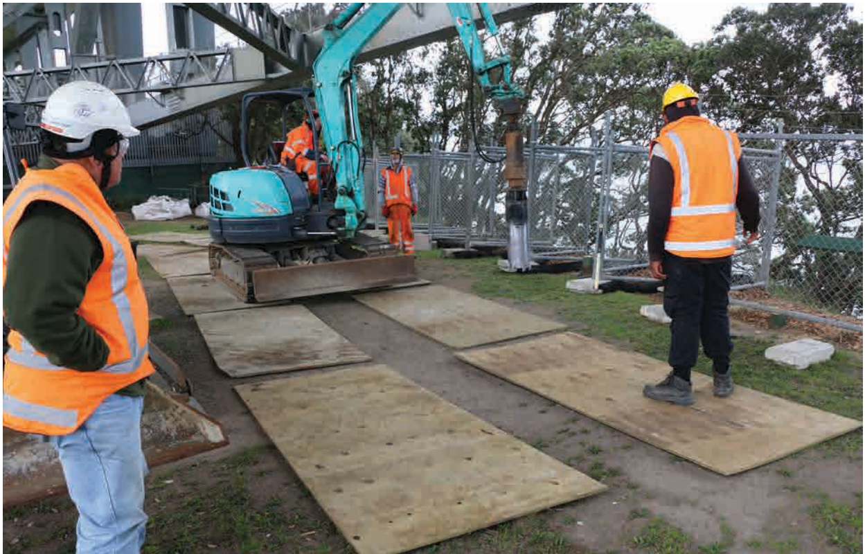
Figure 12. Plywood sheeting being used to mitigate ground disturbance by heavy machinery.
