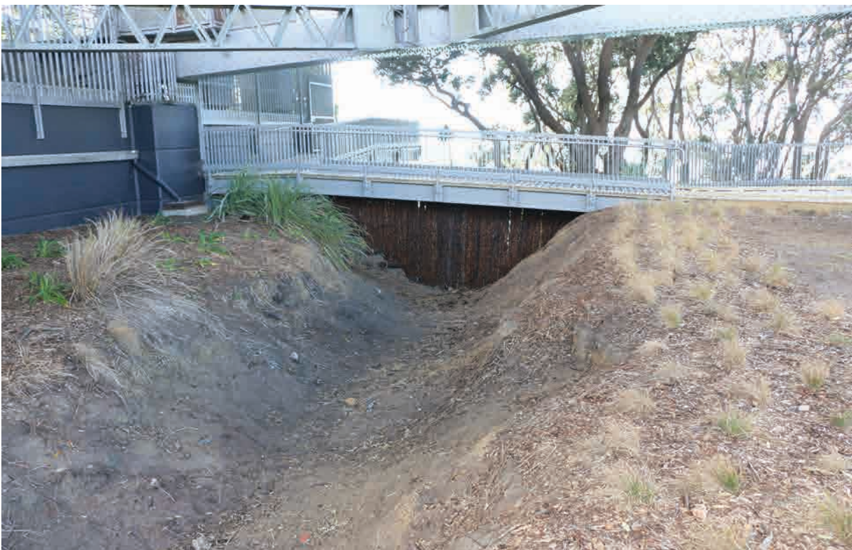
Figure 18. View of vertical ponga underneath foot bridge.
