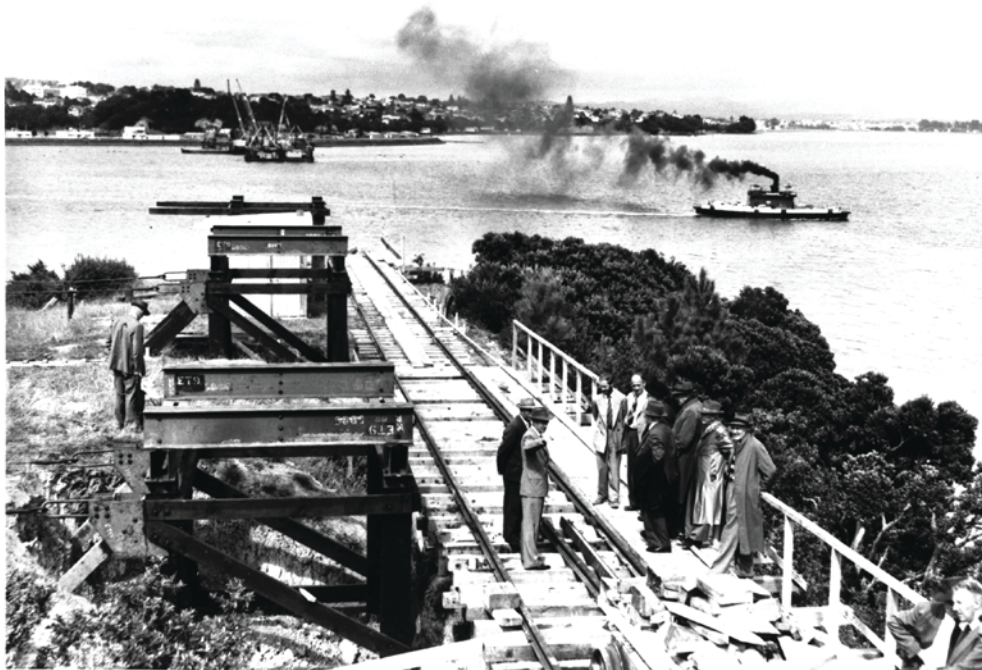
Figure 8 (above). Photo probably dated to 1957 showing the installation of a tramway along the western side of the pa. Note the pier which is being used for support, along with the stays which can be seen presumably attached to anchors to the left of frame. Sir George Grey Special Collections, Auckland Library 459-15.
