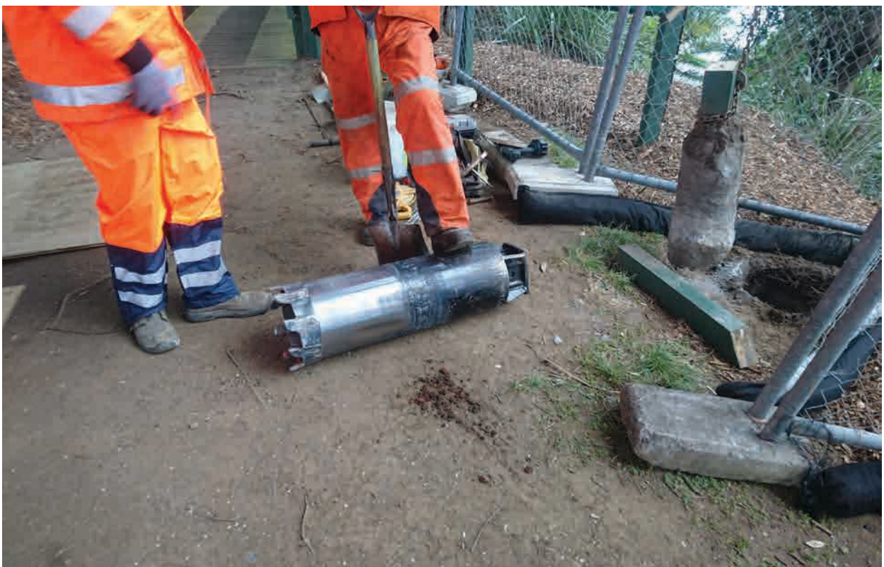
Figure 13. Extracted post and concrete with coring auger.
