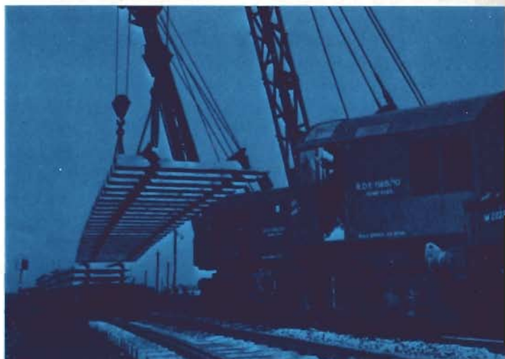
Installing new track layout at Rutherglen.
