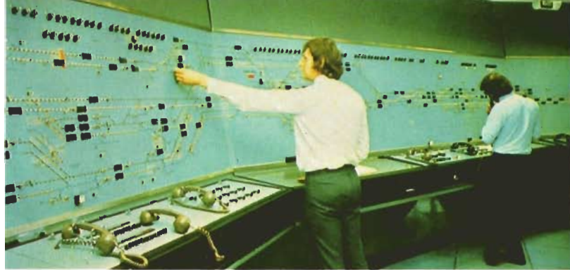
Illuminated diagram Carlisle Power Signal Box.
