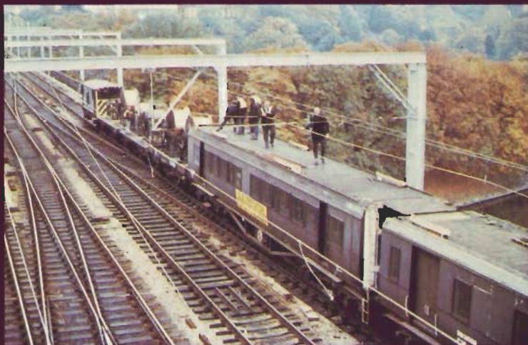
Erecting overhead equipment from a wiring train.
