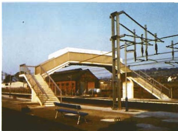
New Footbridge Lockerbie Station.
