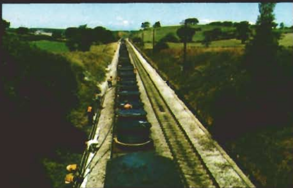
Laying telecommunication cable
