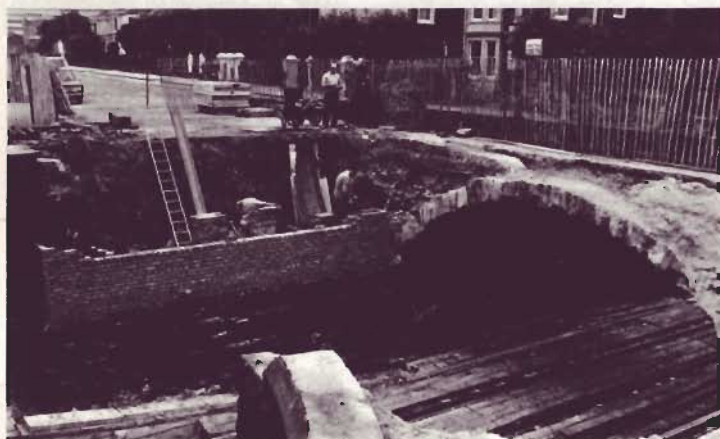
Bridge reconstruction, Scottish Region.
