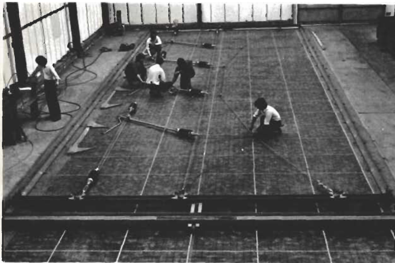
Fabricating headspan wires for overhead equipment.
