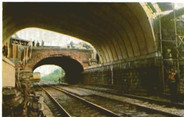
Bridge reconstruction work in progress.
