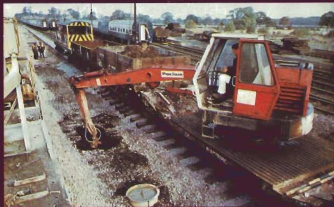
Excavating foundations for lineside structures.
