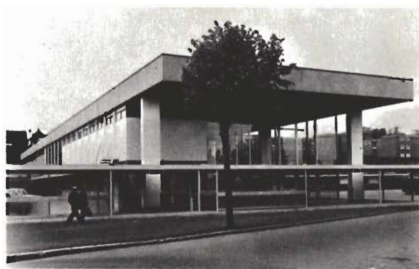
Coventry station re-built during electrification of the line from Birmingham to London.
