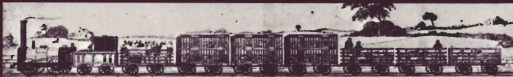
Passenger, Freight and Livestock trains on the Liverpool & Manchester Railway 1837.
