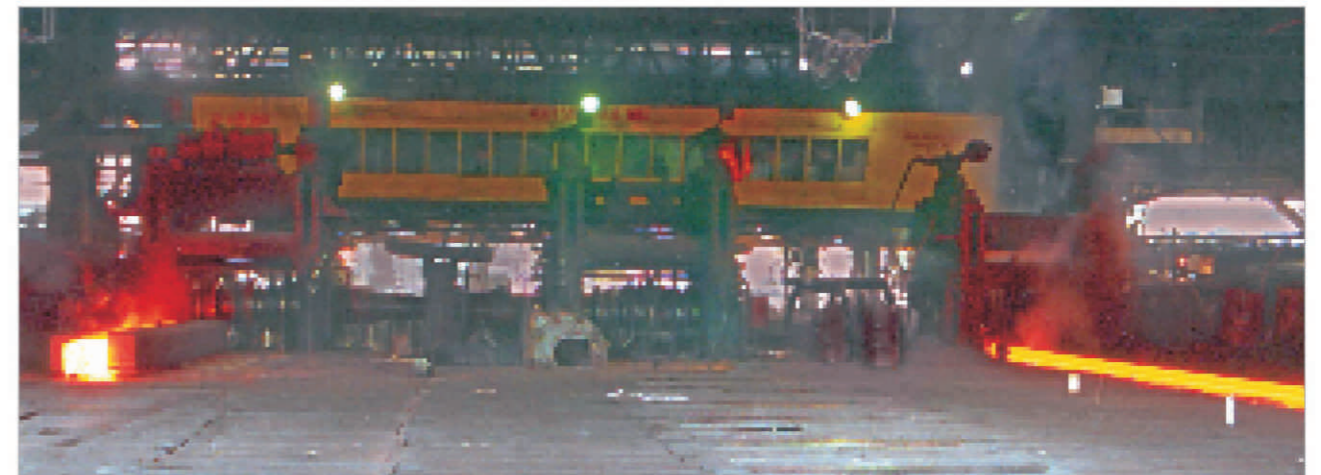
Heavy Structural Mill
