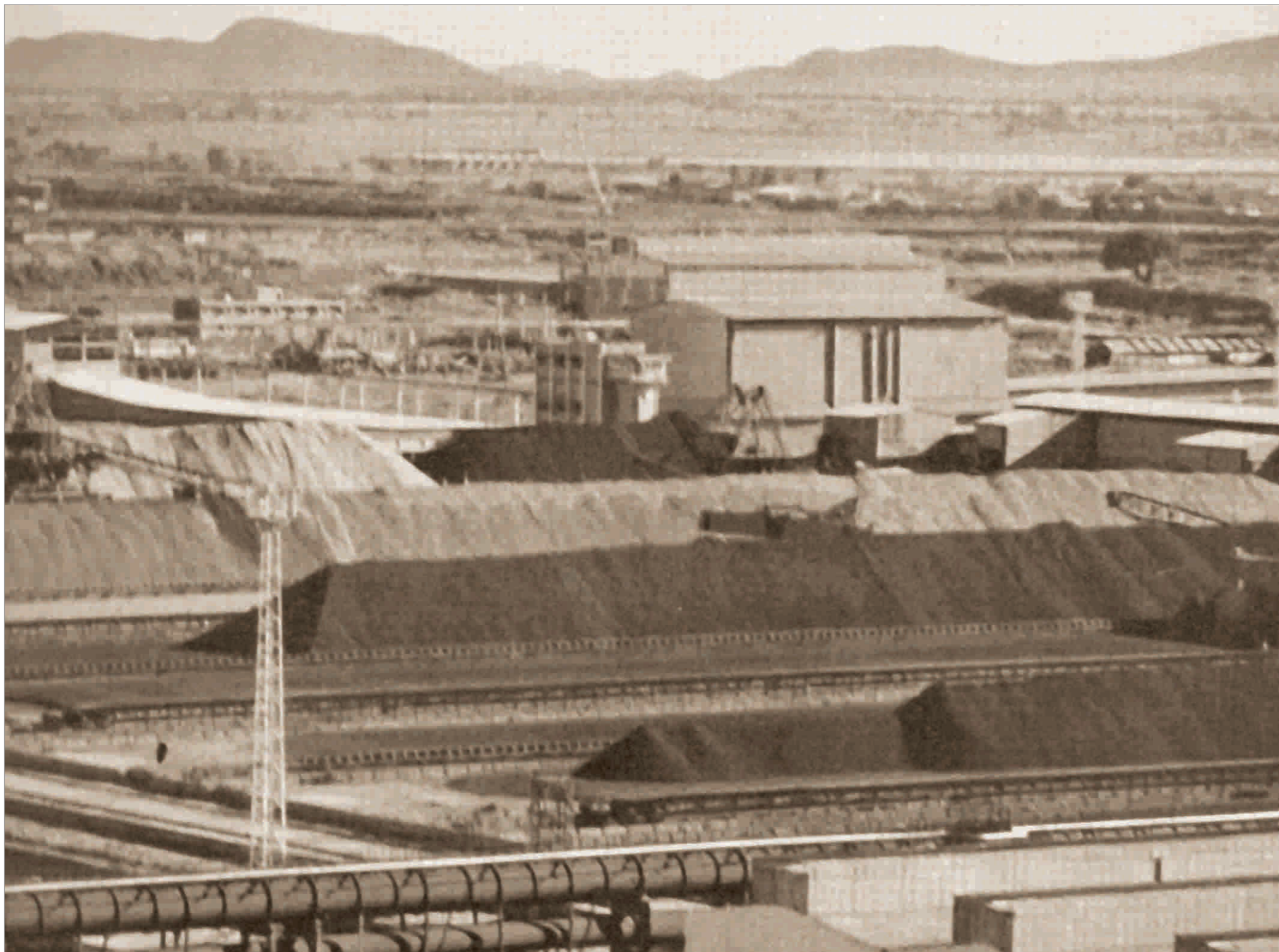
Raw Material Storage and Blending Yard at Bokaro Steel Plant in the late 1970s
