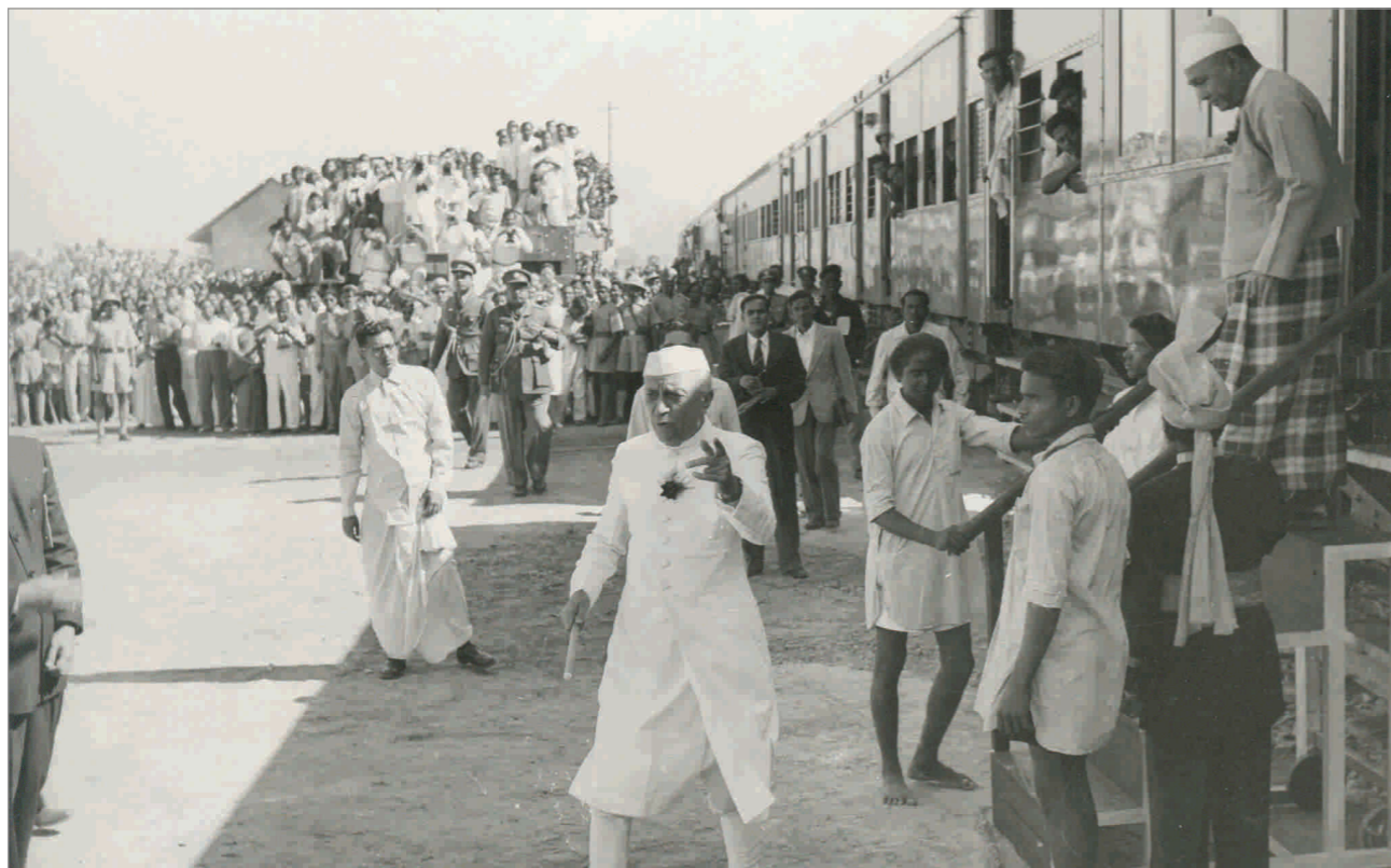
1957: Pandit Nehru alighting from a train at Rourkela Steel Plant. Premier U Nu of Burma accompanied him on this visit
