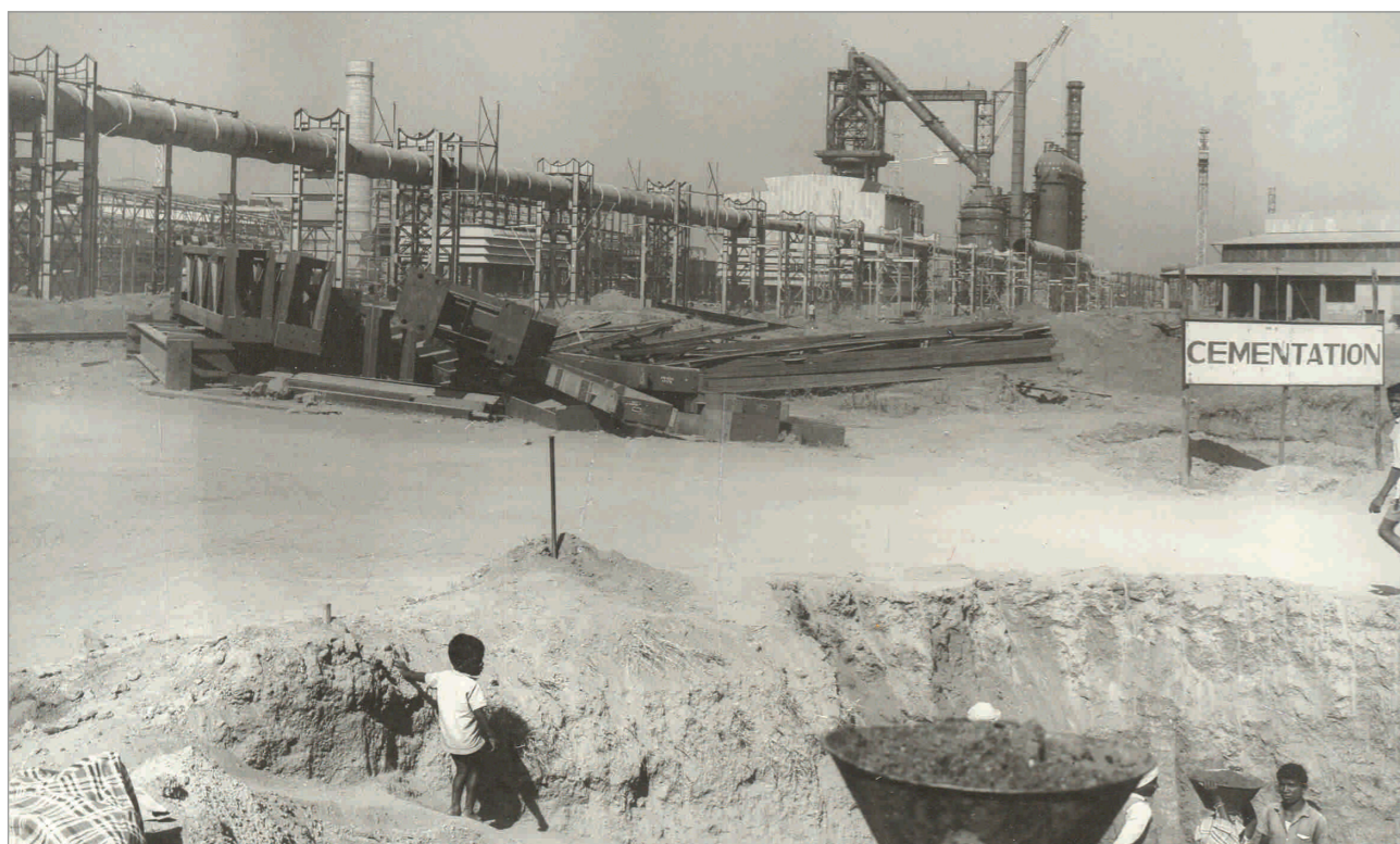
Construction work of Bokaro Steel Plant in progress
