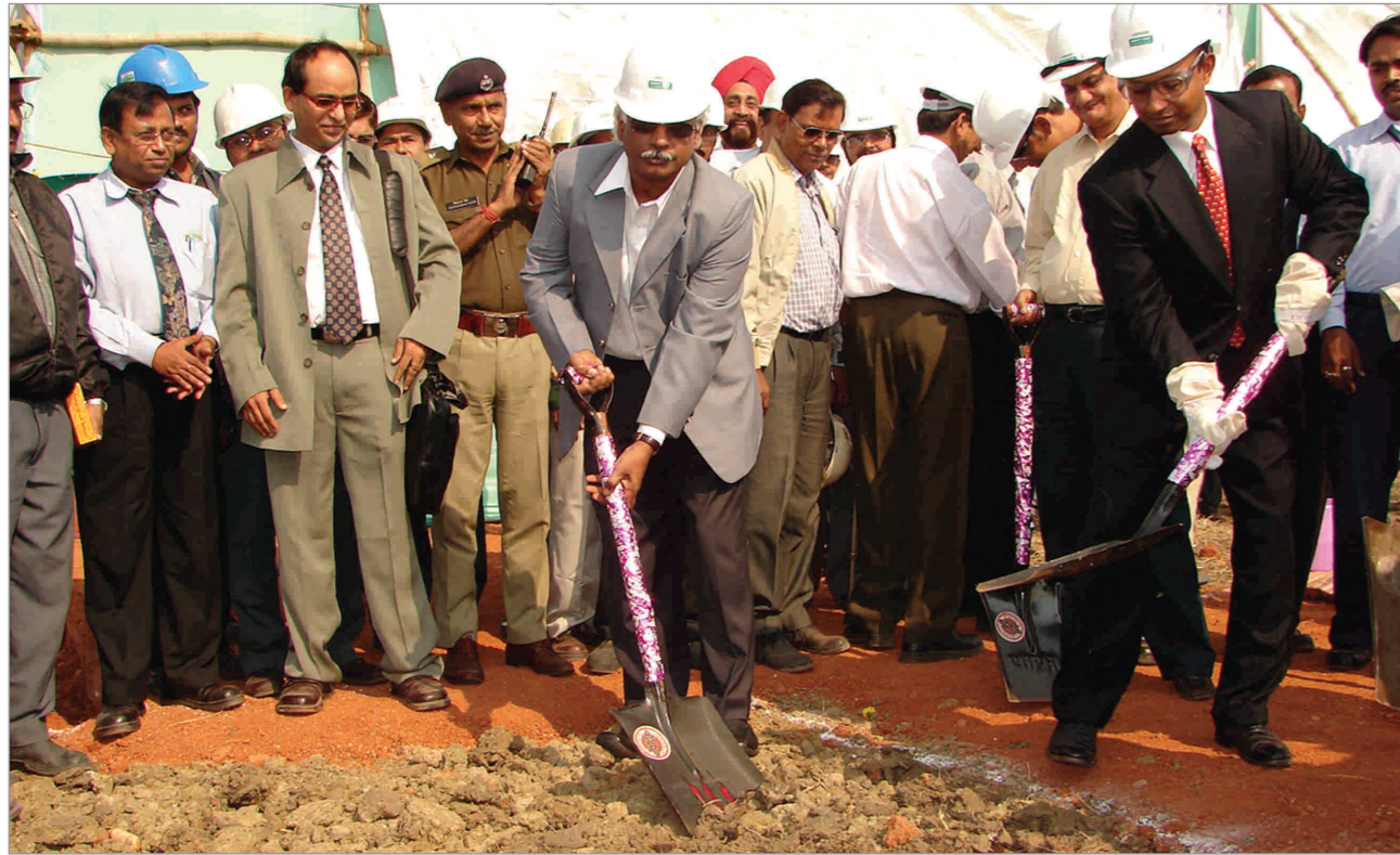
Mr V Shyamsundar, Managing Director, breaks ground for a 700 MTPD air separation unit coming up at Durgapur Steel Plant
