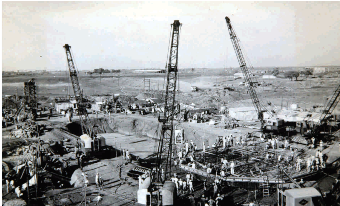
June, 1957: Concreting of Blast Furnace # 1 of Bhilai
