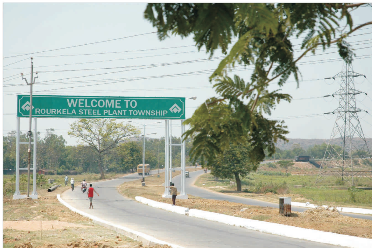
Road to township
