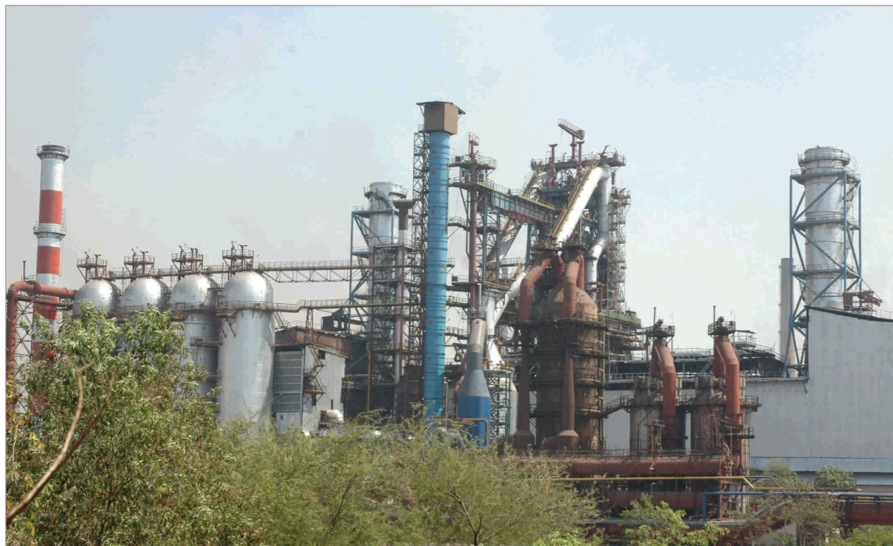
Blast Furnace # 7 of Bhilai Steel Plant after technological upgradation
