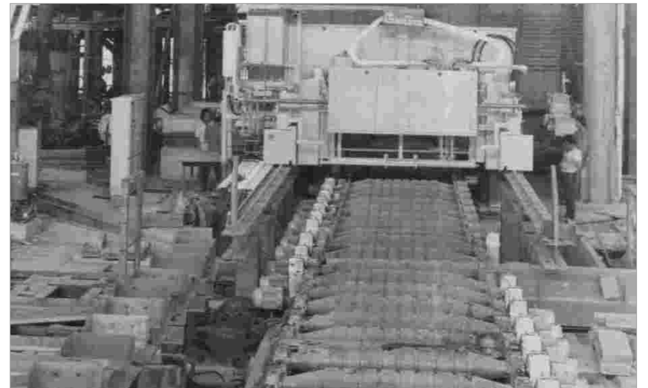
May, 1982: View of the Bloom-cum-Slab Mill during the Stage I expansion of Alloy Steels Plant
