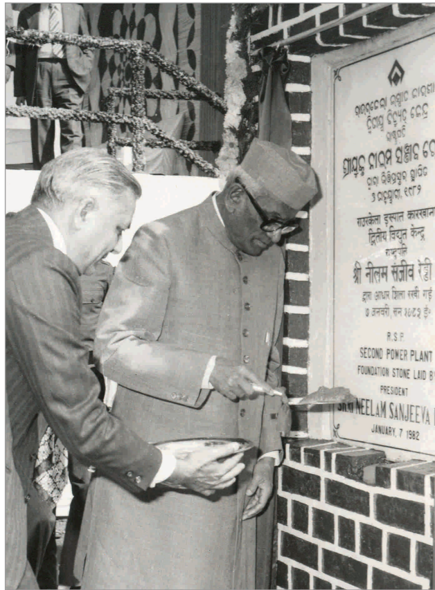
January 2, 1982: President Shri Neelam Sanjeeva Reddy laying the foundation stone of the second captive power plant of Rourkela Steel Plant
