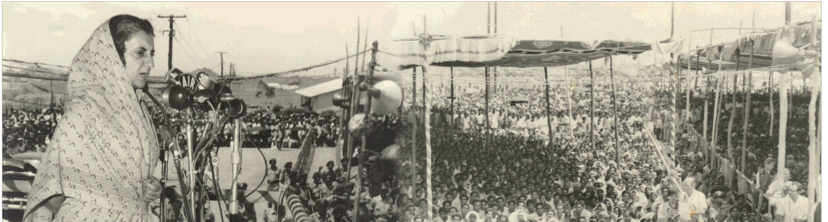
April 6, 1968: Prime Minister Smt Indira Gandhi addressing a gathering on the occasion of concrete pouring of the first blast furnace of Bokaro Steel Limited
