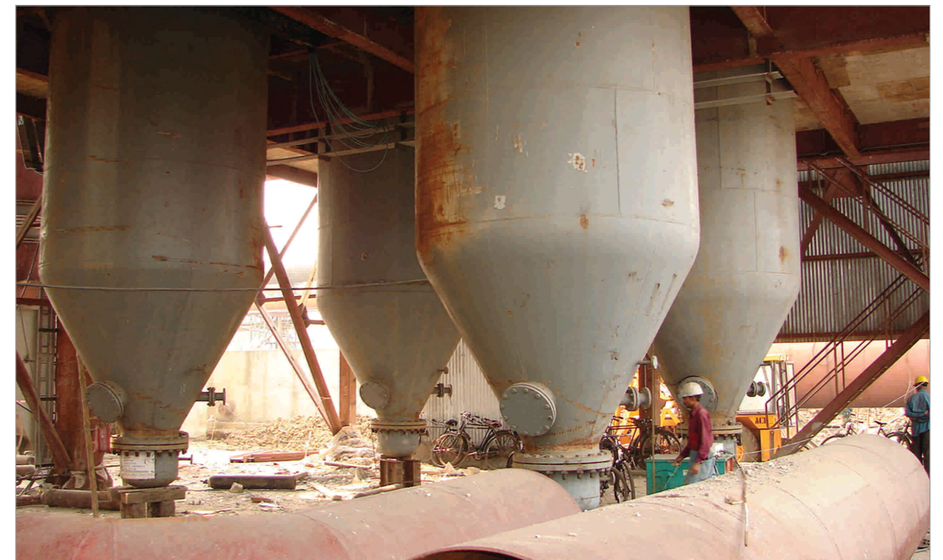
Coal dust injection plant under construction at Durgapur Steel Plant
