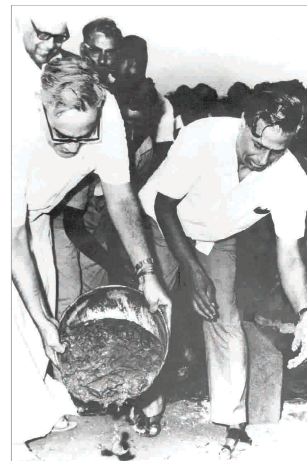
June 13, 1972: Shri Mohan Kumaramangalam, Steel Minister, inaugurating construction of Salem Steel Plant
