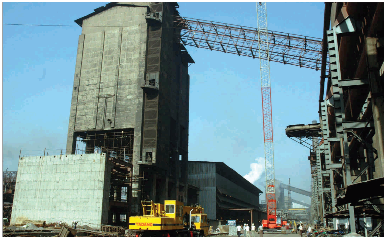
Rebuilding of Coke Oven Battery # 5 of Bhilai Steel Plant under progress
