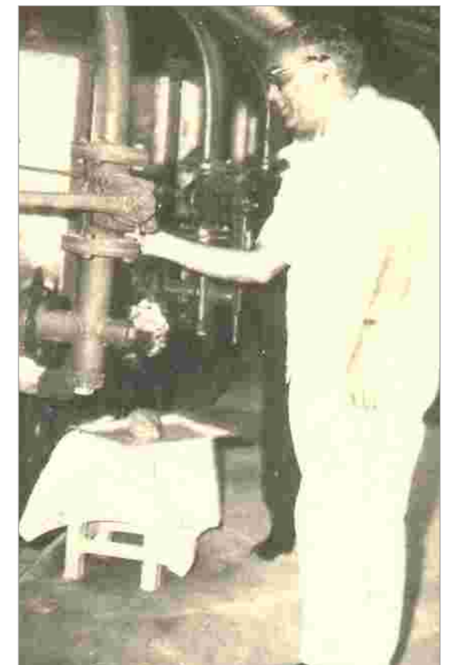
Steel Minister Shri Mohan Kumaramangalam inaugurated a coke oven battery at Bokaro Steel Plant on September 9, 1972
