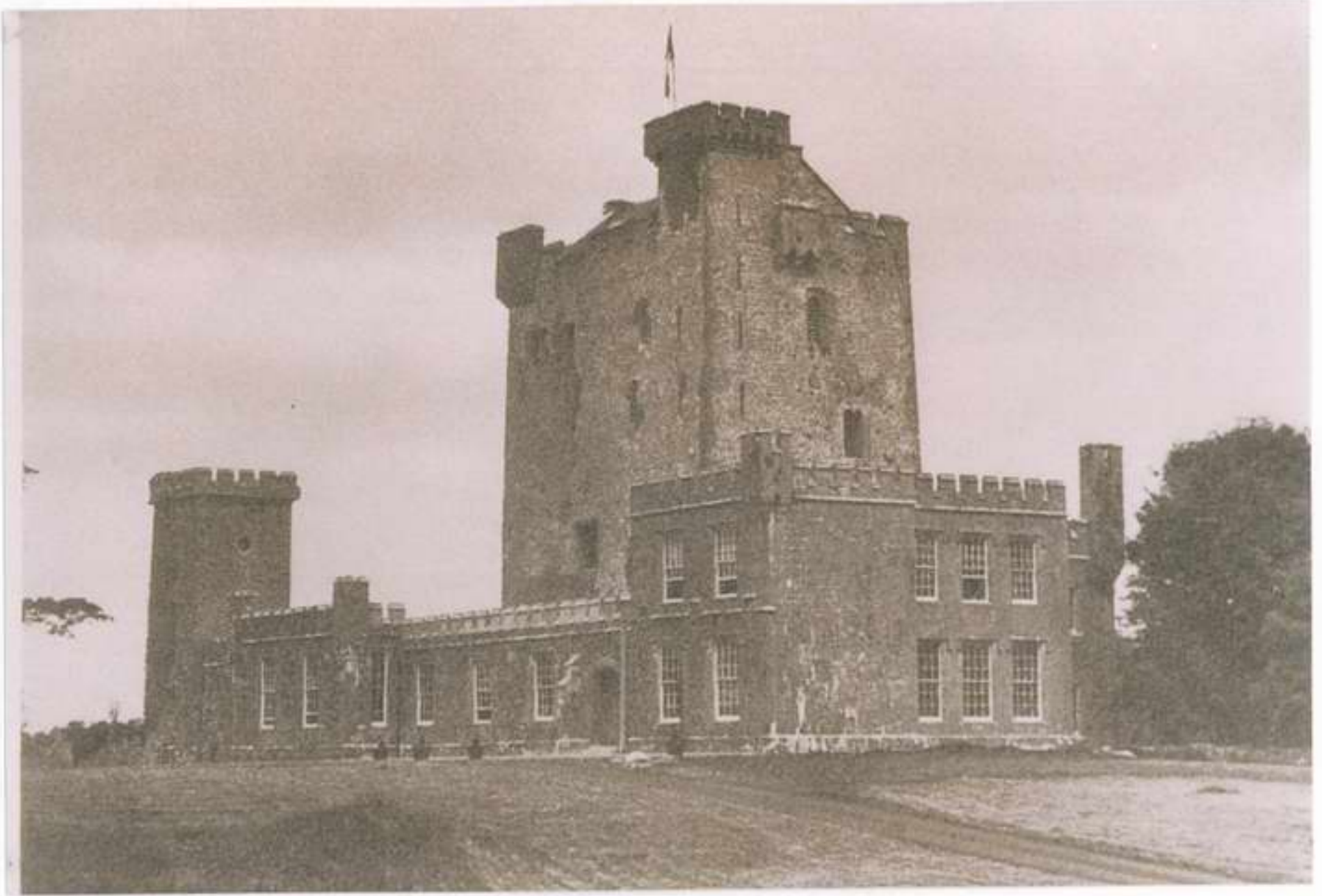
Fig. 45 Knappogue Castle, Co. Clare. Late medieval tower house with nineteenth century castellated range believed to be by James Pain.
