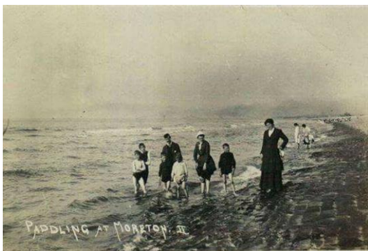
The Leasowe ‘Breakwater’ at Moreton.
