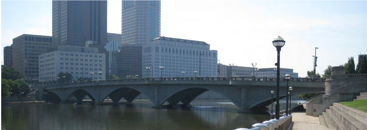
Photo 8-4. Broad Street Bridge looking south
