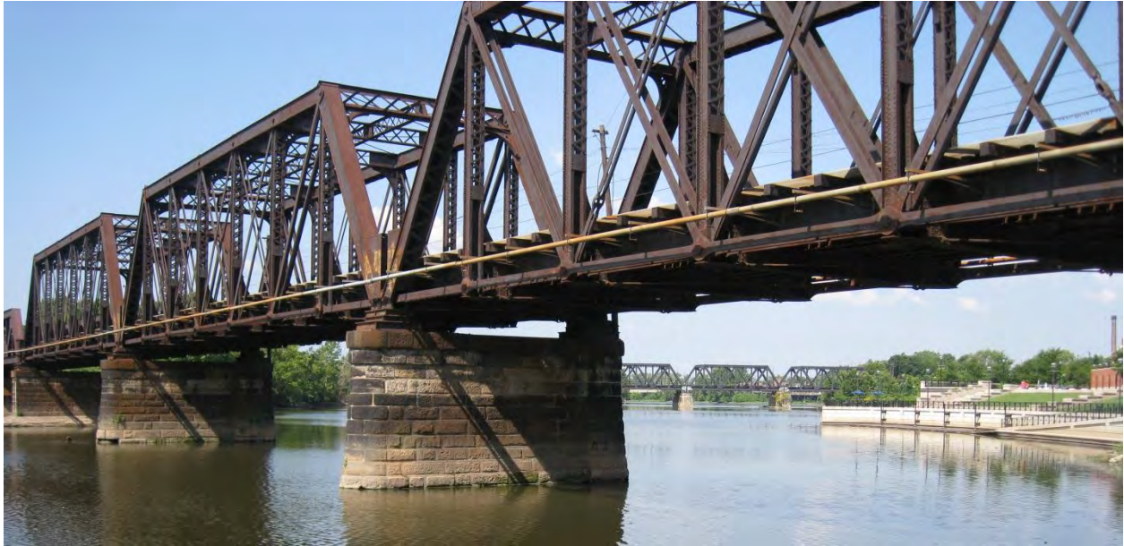
Photo 8-5. Norfolk Southern and CSX Bridges (looking north)
