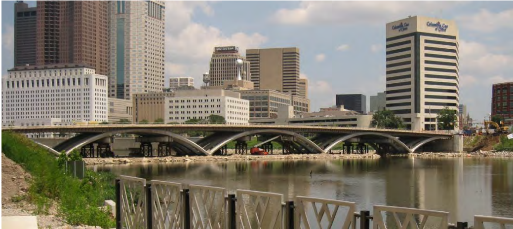
Photo 8-3. Rich Street Bridge looking north
