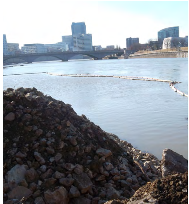
Containment booms installed
