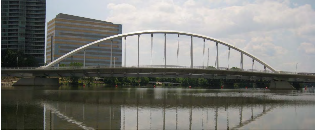
Photo 8-2. Main Street Bridge (looking south)
