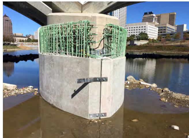
Bridge skirt installation
