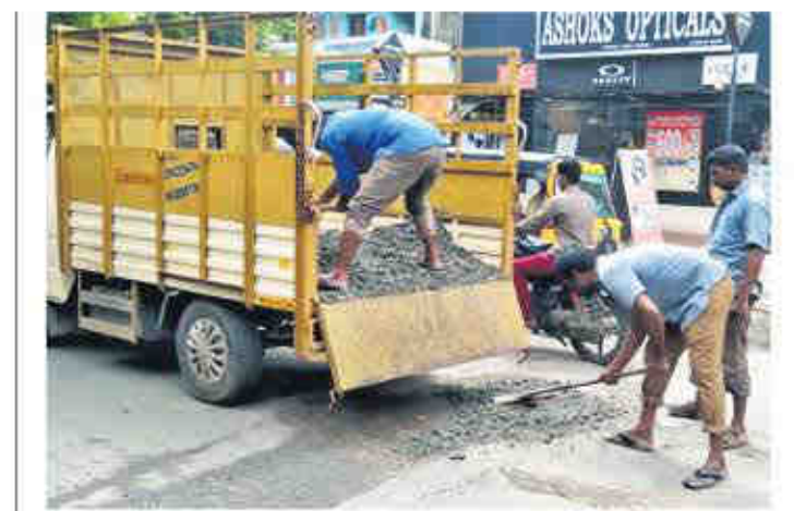
Workers patching up potholes on a road in the city | SPECIAL ARRANGEMENT
