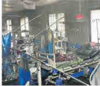
Charred remains at the Ahmednagar hospital ICU after the fire | PTI
