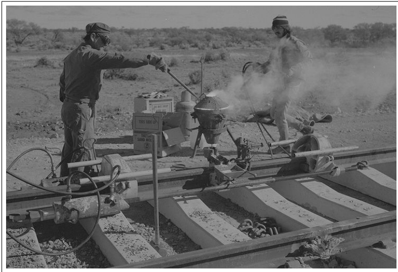
Building the Tarcoola to Alice Springs line ( NRM Collection )
