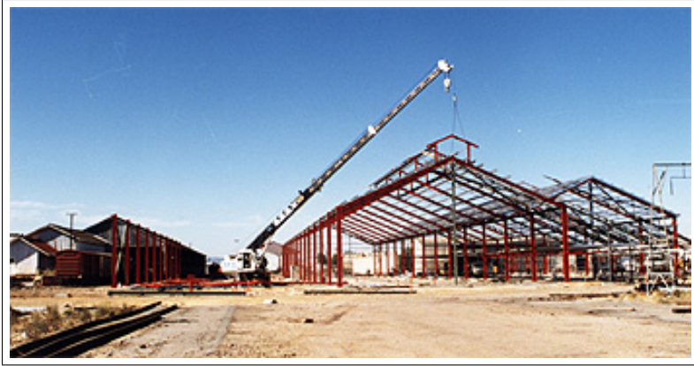
The current museum under construction ( NRM Collection )
