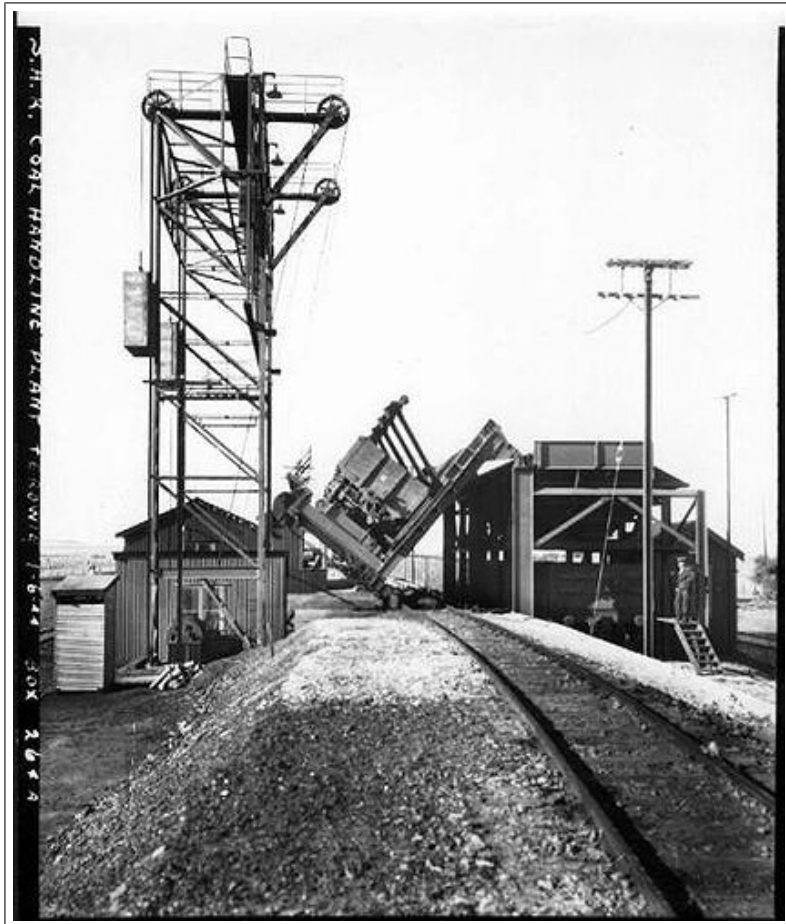
Transferring coal from narrow gauge wagons to broad gauge wagons at Terowie ( NRM Collection )
