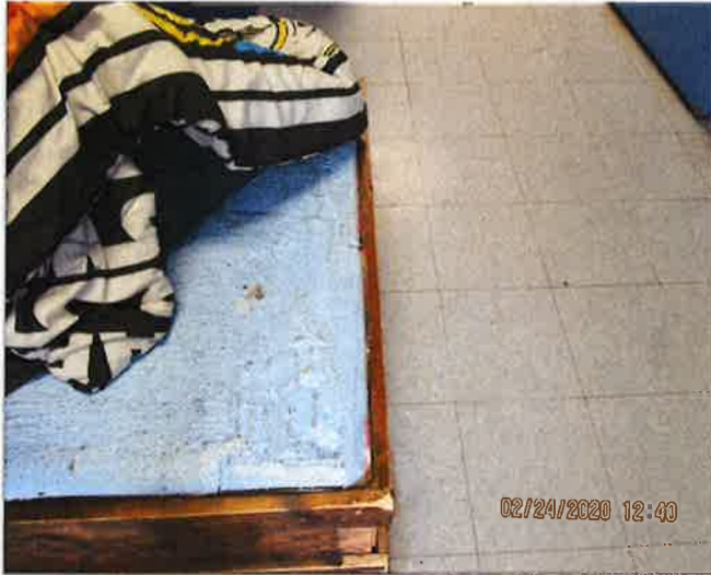
Figure 2 Concrete bed slab
