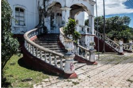
Fig. 11. The appearance of the abandoned mansion.
