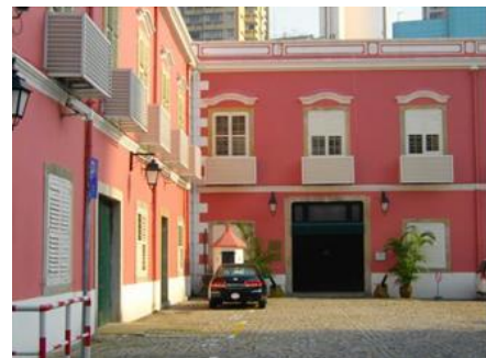
Fig. 3. One corner of the office building of the Macau Security Forces Command.
