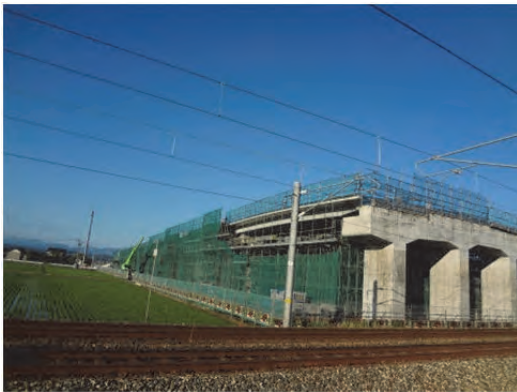
Figure 5.1.6 Example of Fixed Supporting Method
