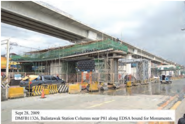
Figure 5.1.7 Station Construction – LRT Line 1 NEP
