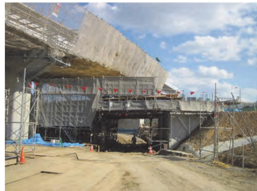
Figure 5.1.6 Example of Fixed Supporting Method
