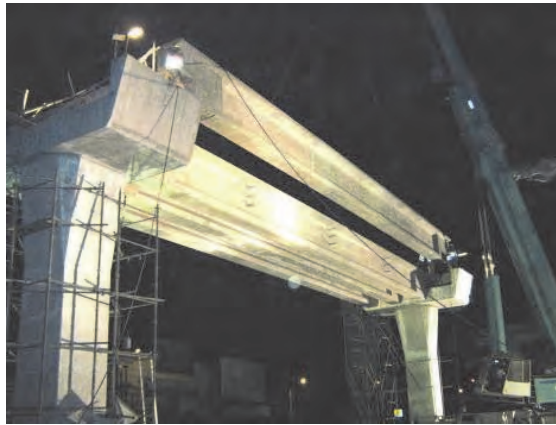
Figure 5.1.5 Girder Erection by Single Truck Mounted Crane – LRT Line 1 NEP
