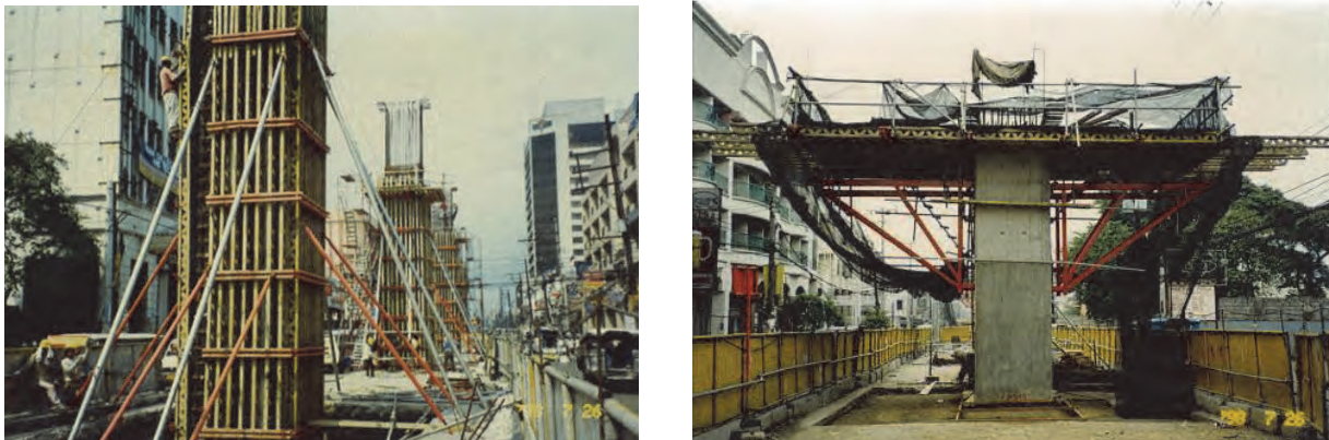
Figure 5.1.2 Pier Column Construction – LRT Line 2
